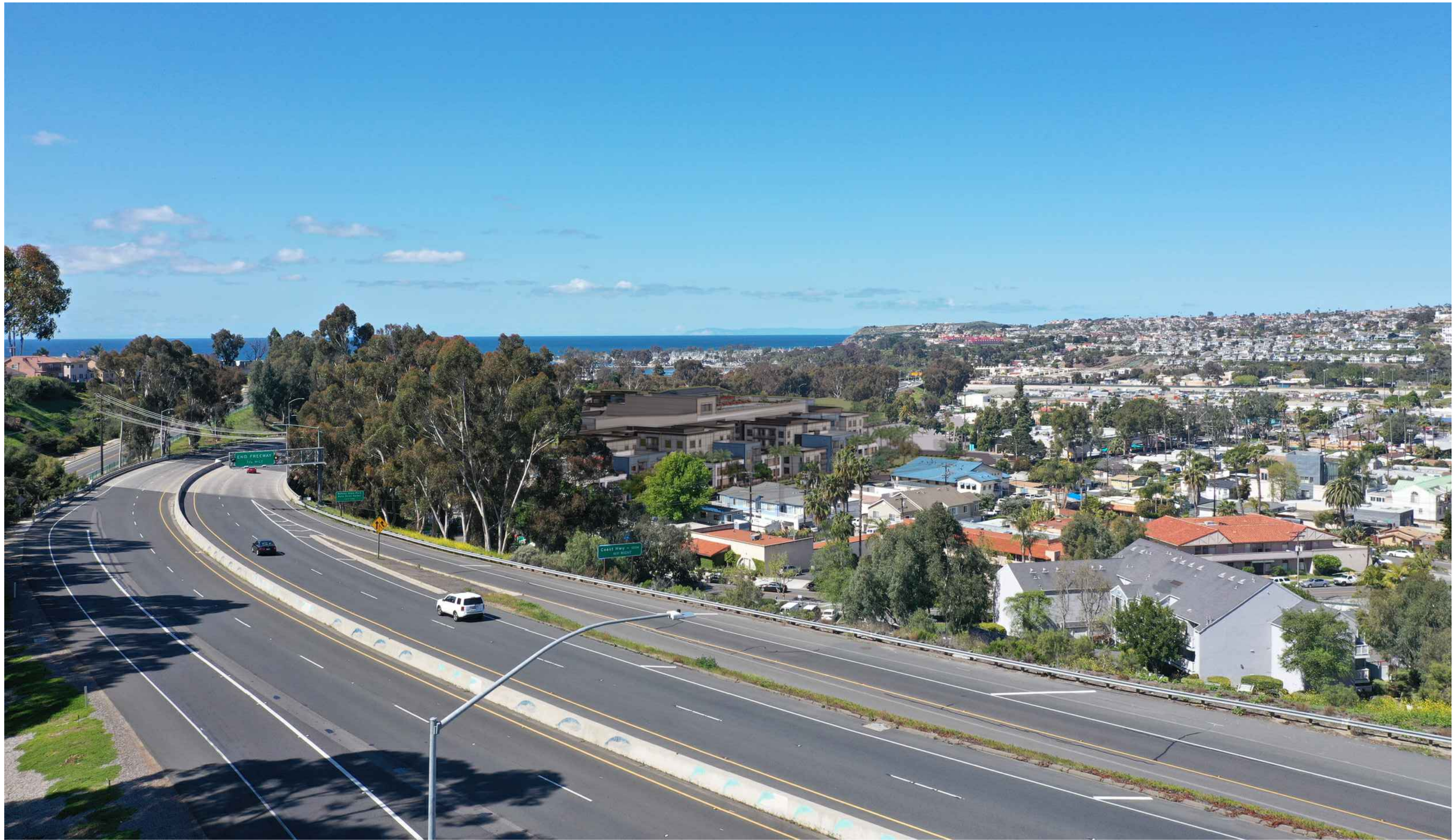
View from Off-Ramp Facing West
