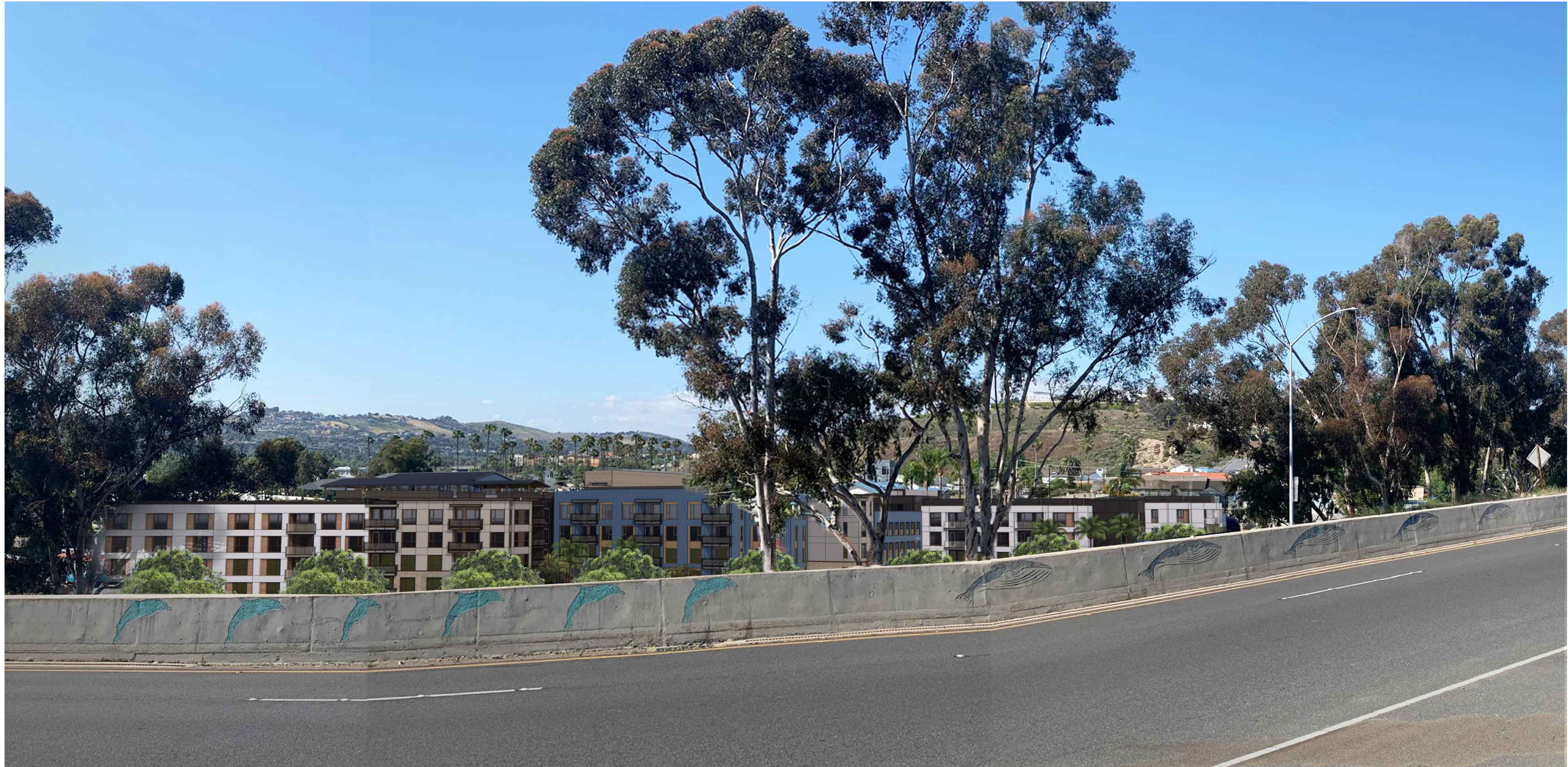
View from Off-Ramp Facing North towards the Rear elevation of the Project
