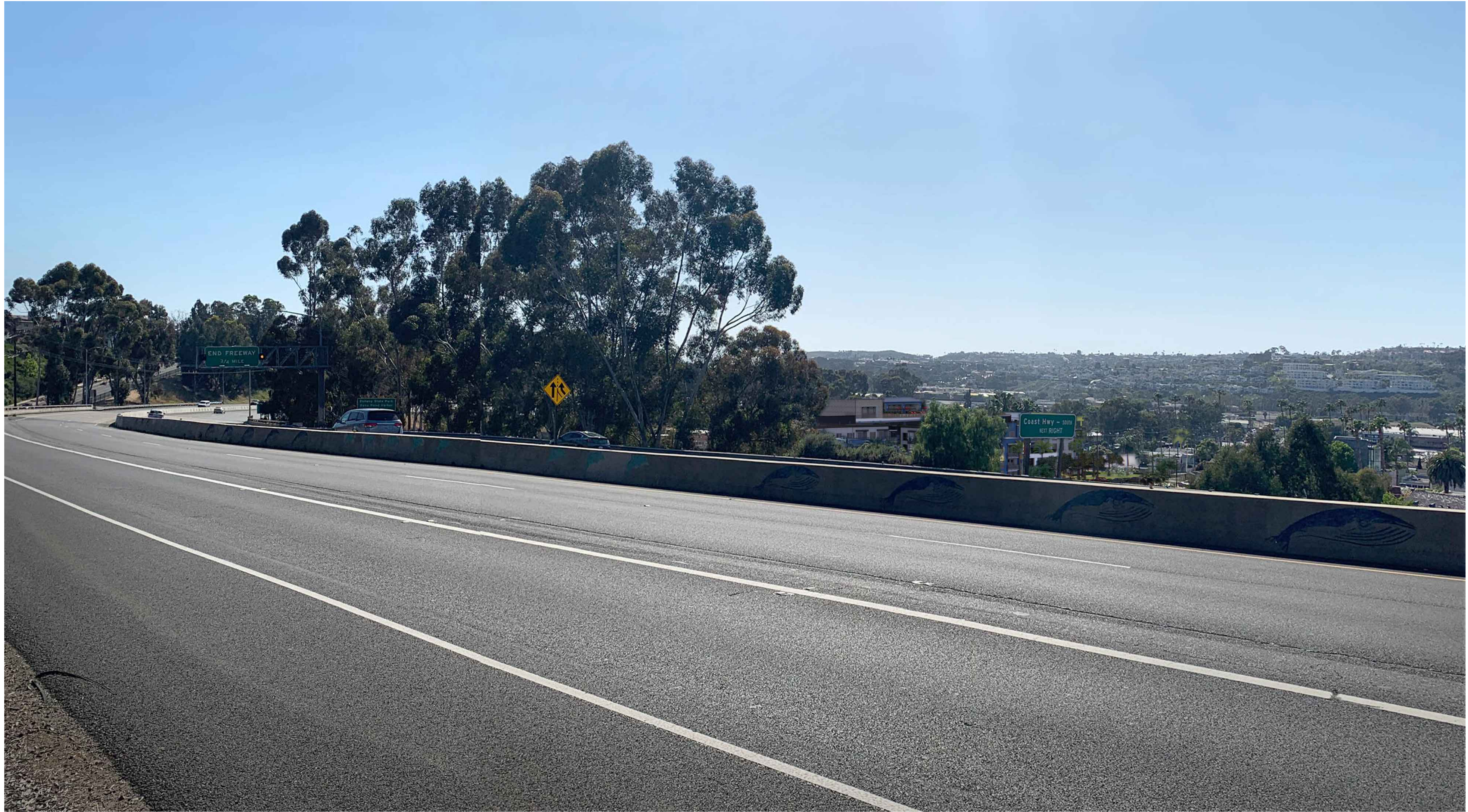
View from Off-Ramp Facing West
