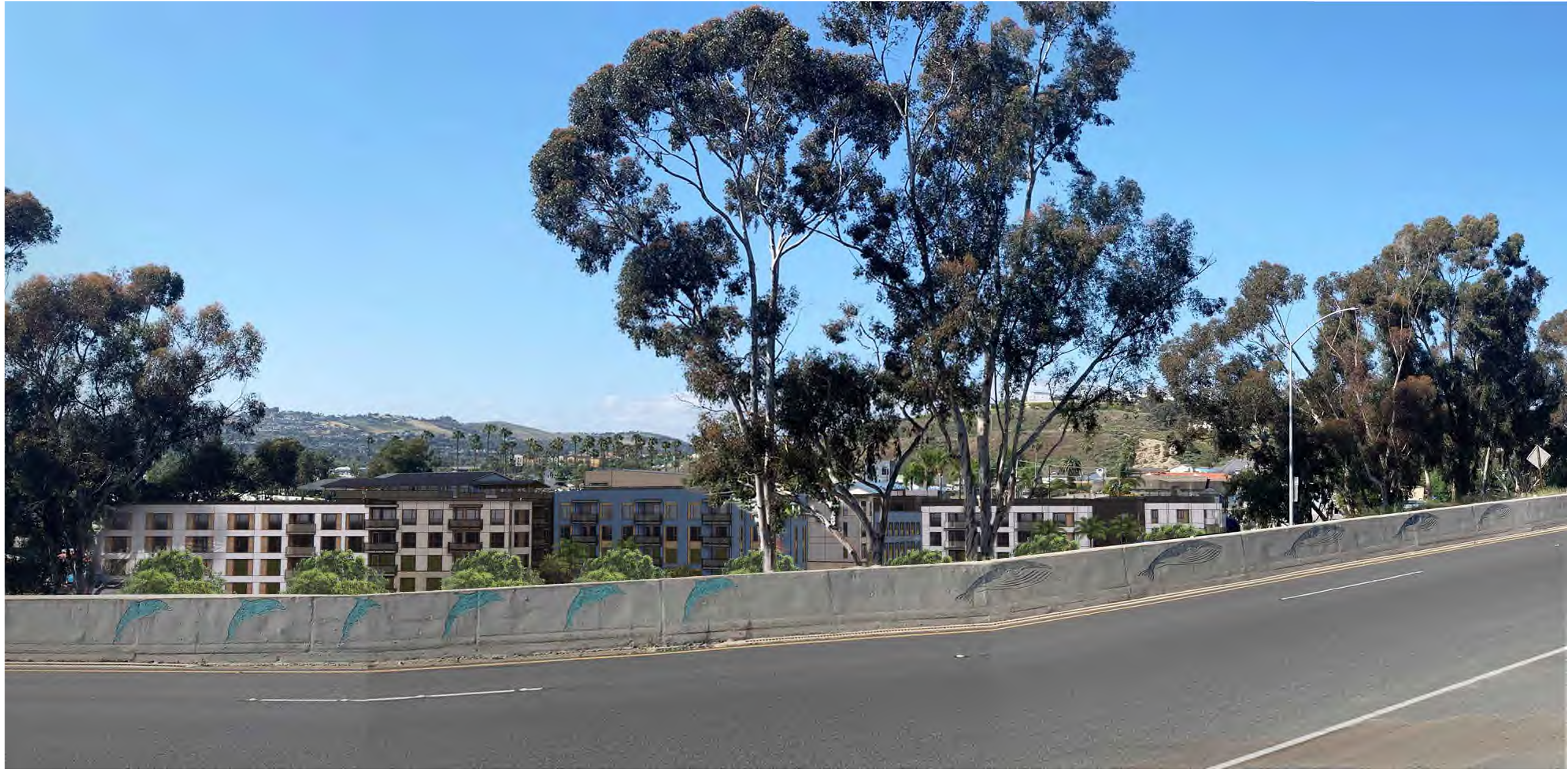
View from Off-Ramp Facing North towards the Rear elevation of the Project
