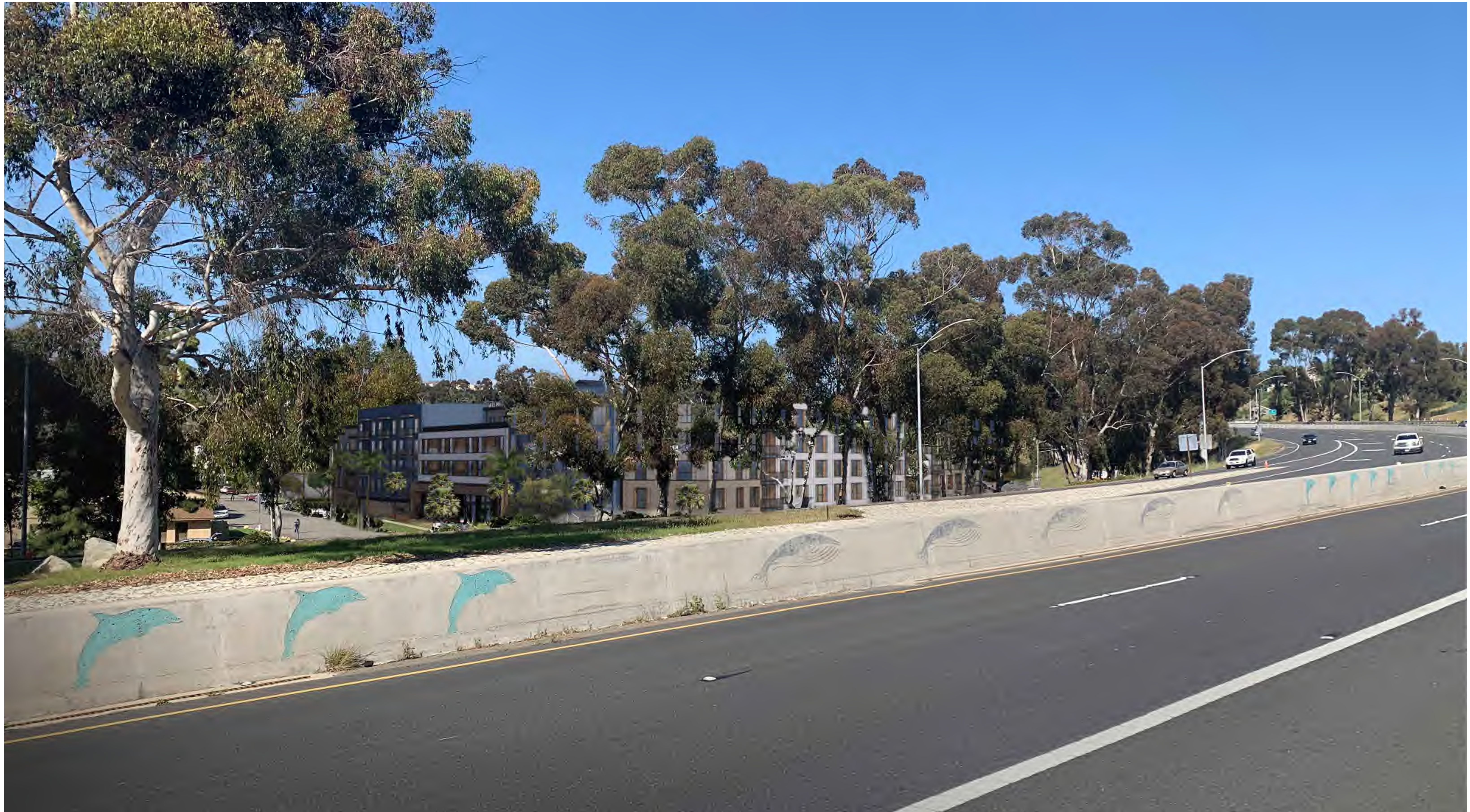
View from Off-Ramp Facing East towards the corner of Sepulveda and the Proposed E.V.A.
