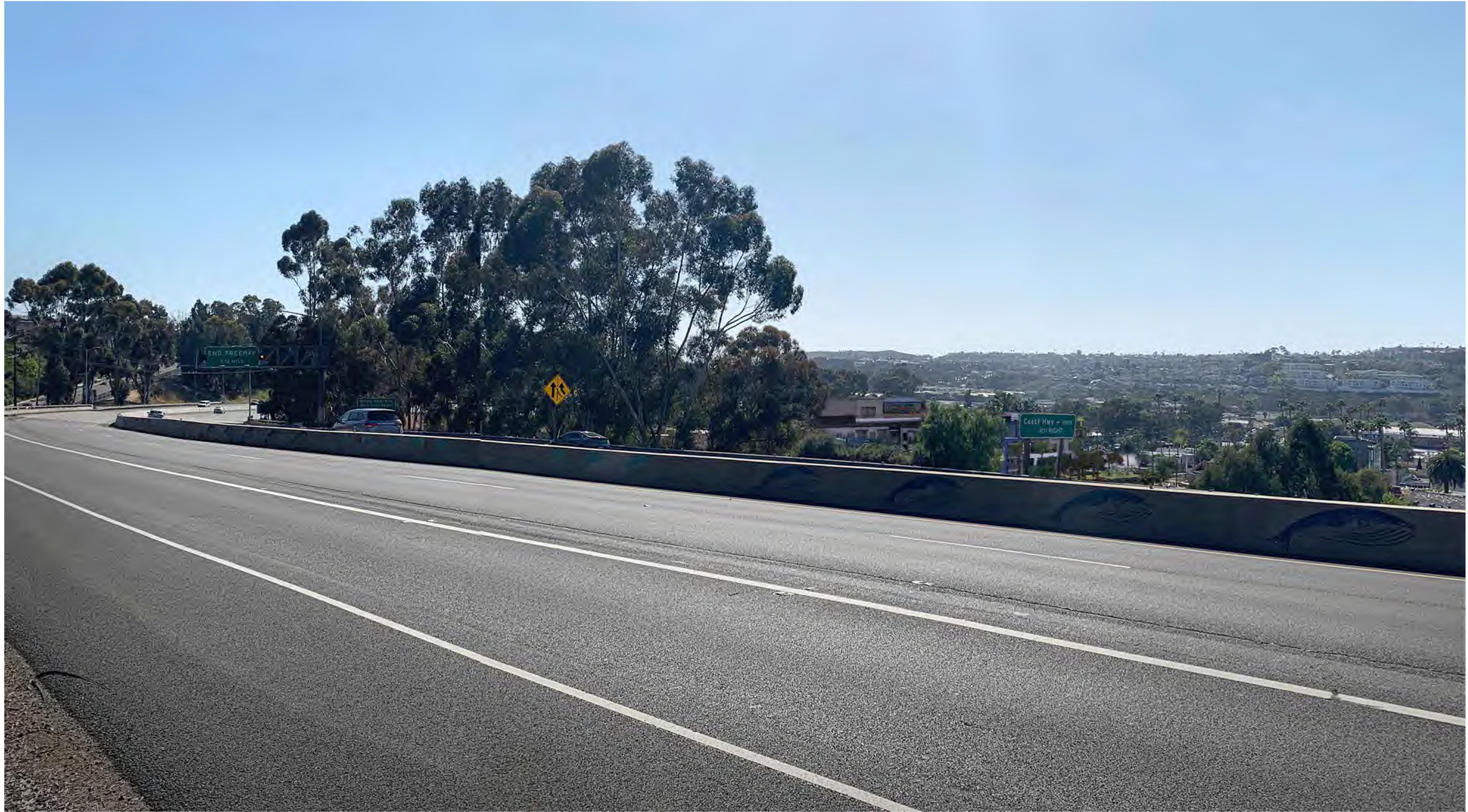
View from Off-Ramp Facing West
