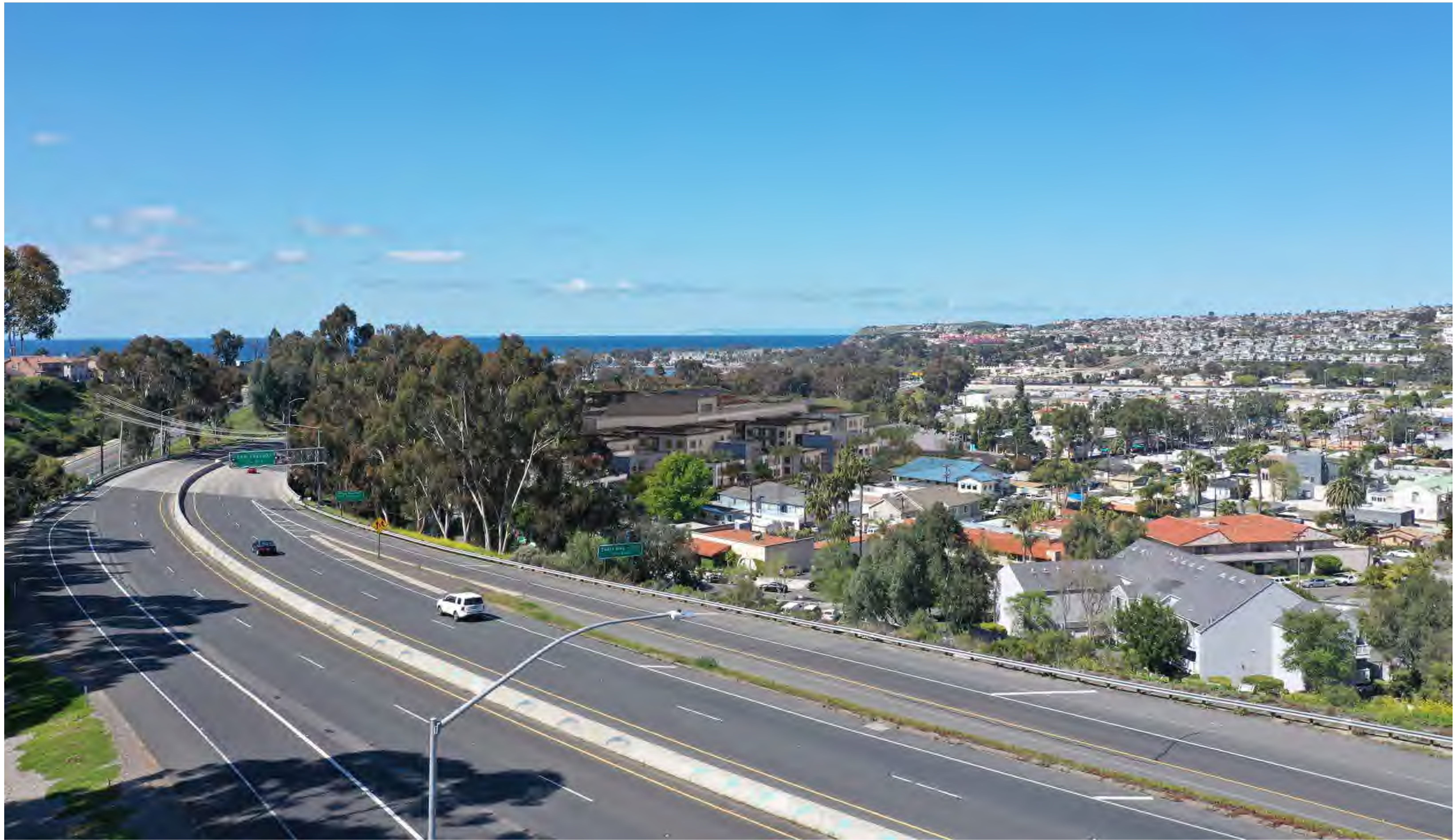
View from Off-Ramp Facing West
