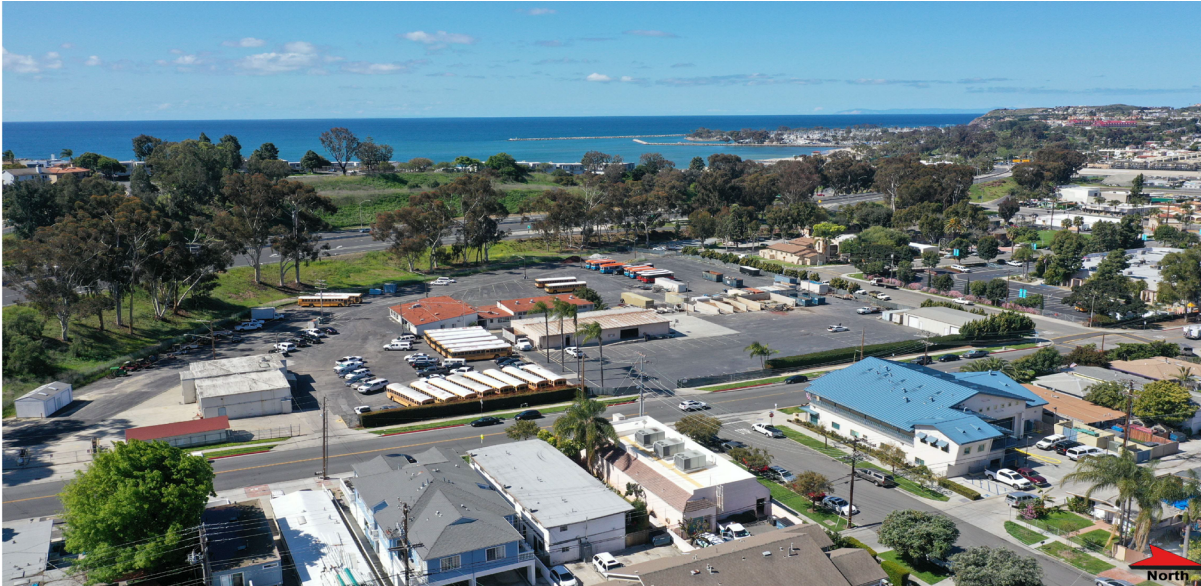
Aerial View of Project Site from adjacent eastern properties across Victoria Blvd
