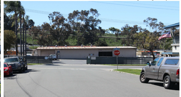
View of Victoria Blvd from Via Santa Rosa
