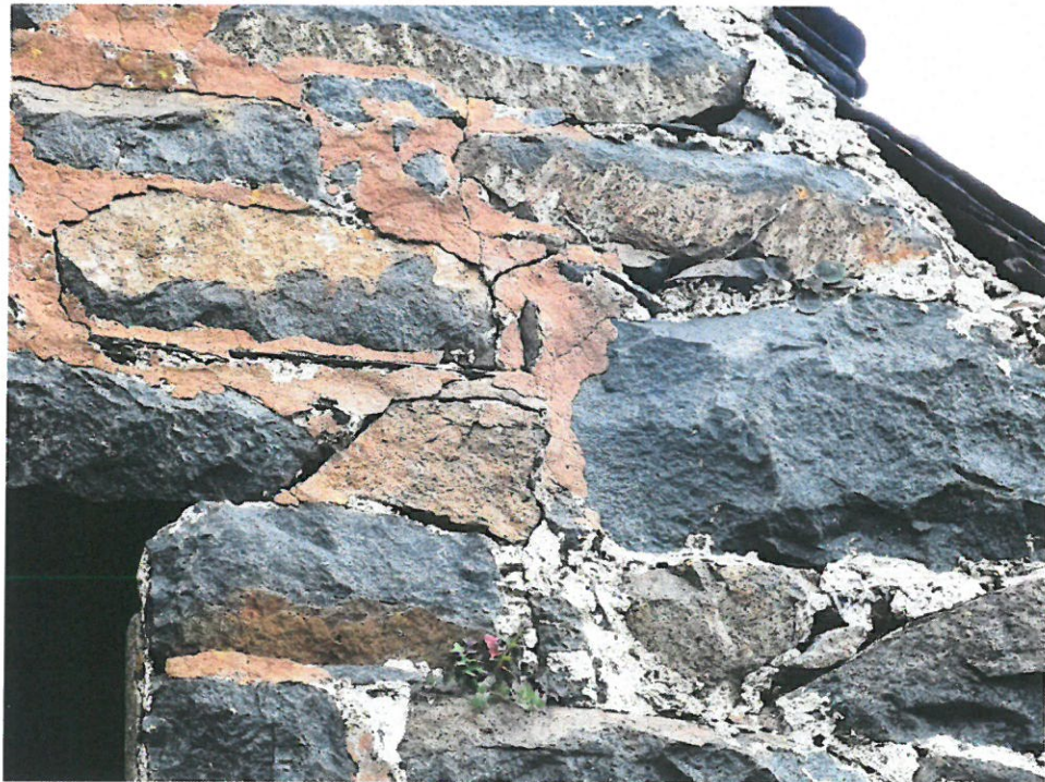
South-West Elevation – Area B – Vertical Cracking
