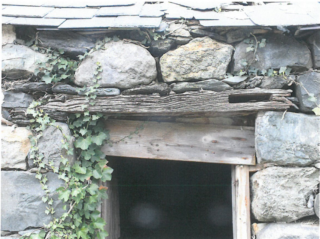
6 South-East elevation – Area C – Door Lintel
