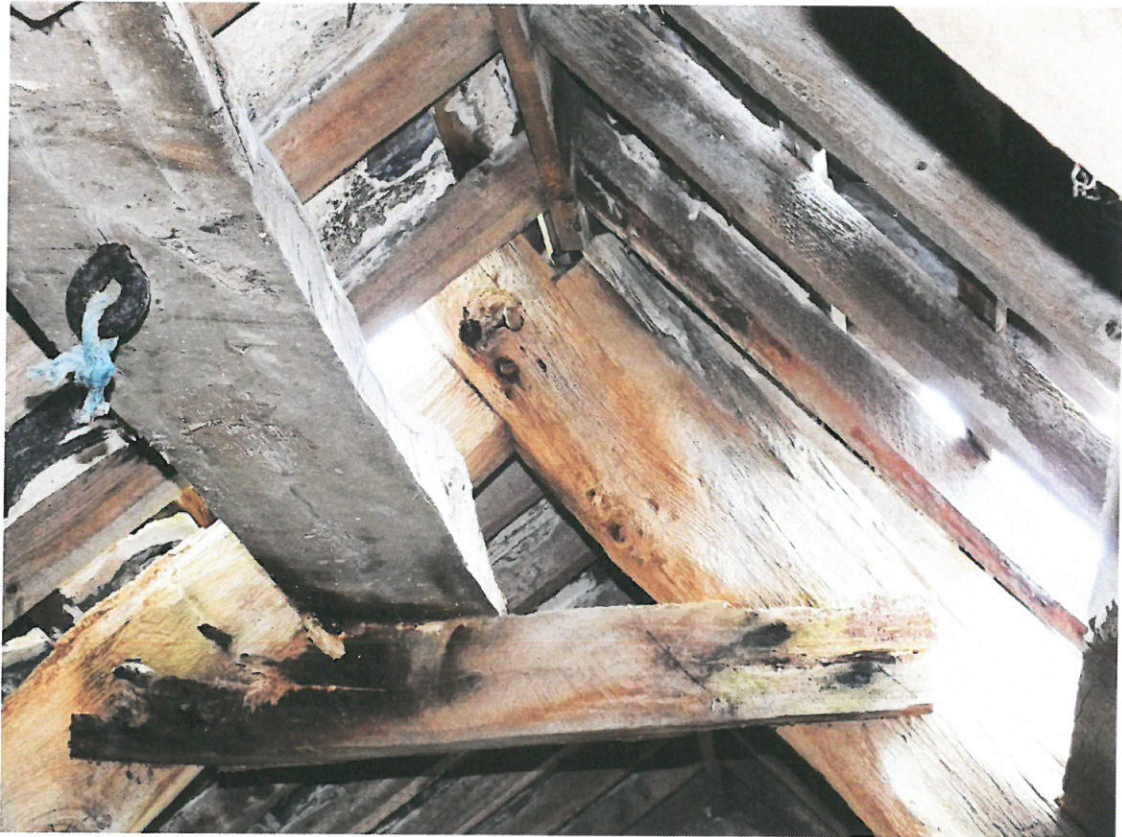
32 Area A – Truss 1
