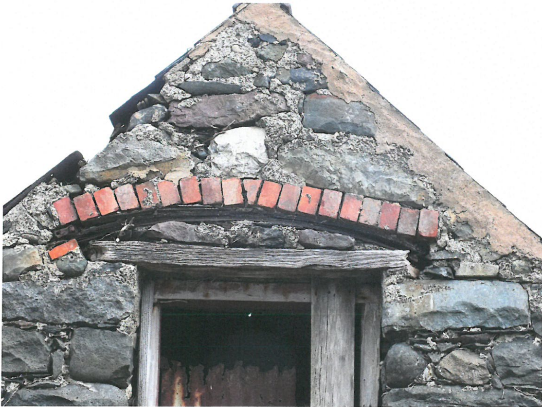
12 South-West Elevation – Area C – Door Lintel
