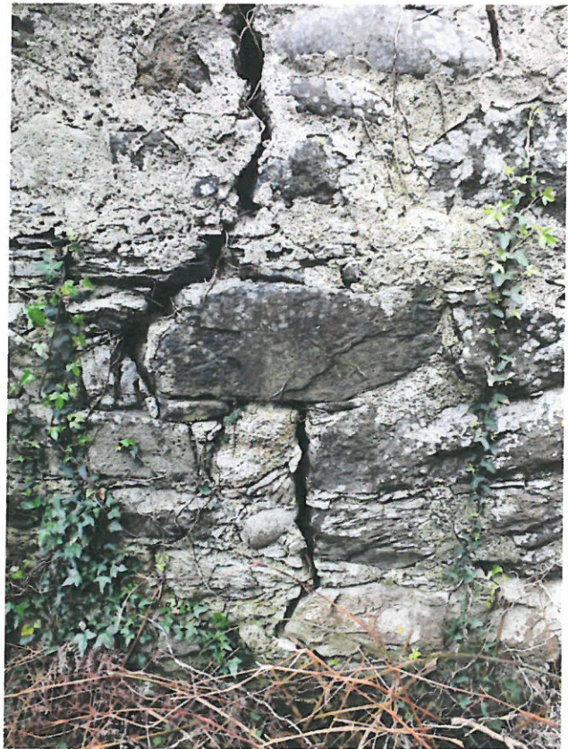
North-East Elevation – Area A – Vertical Crack
