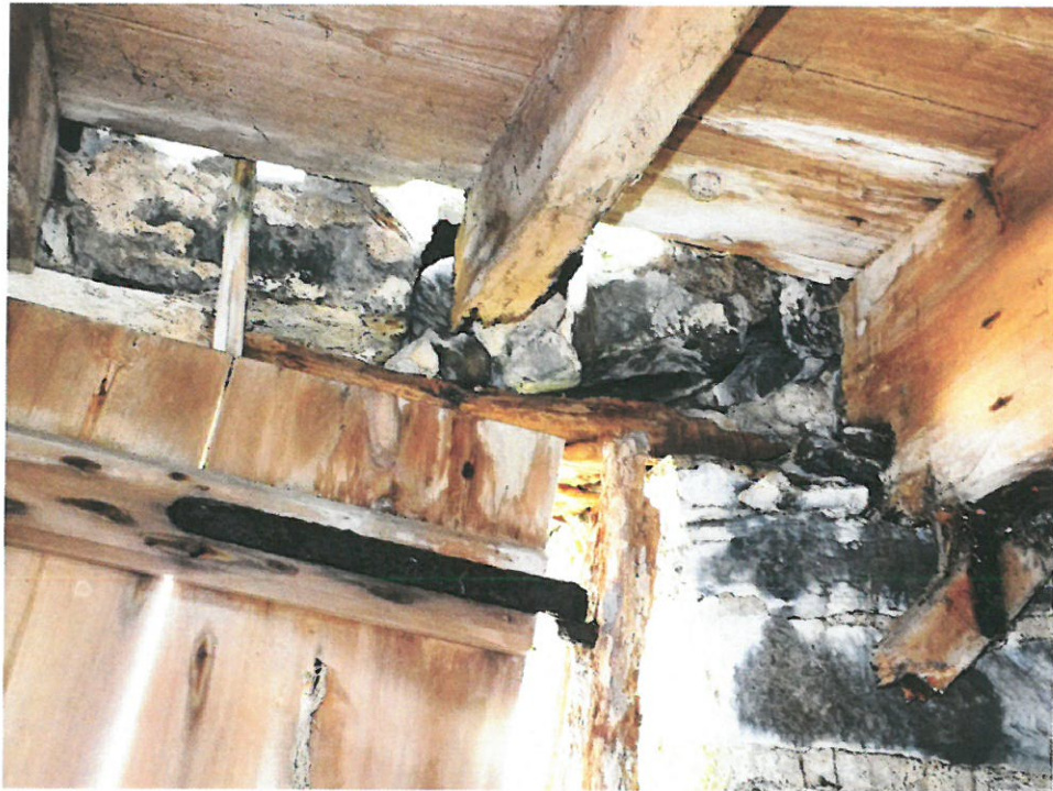
Area B – Vertical Crack in North-West Wall
