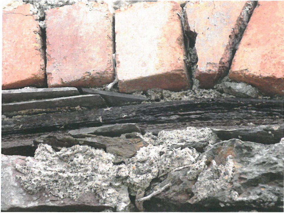
South-West Elevation – Area C – Corroded Plate
