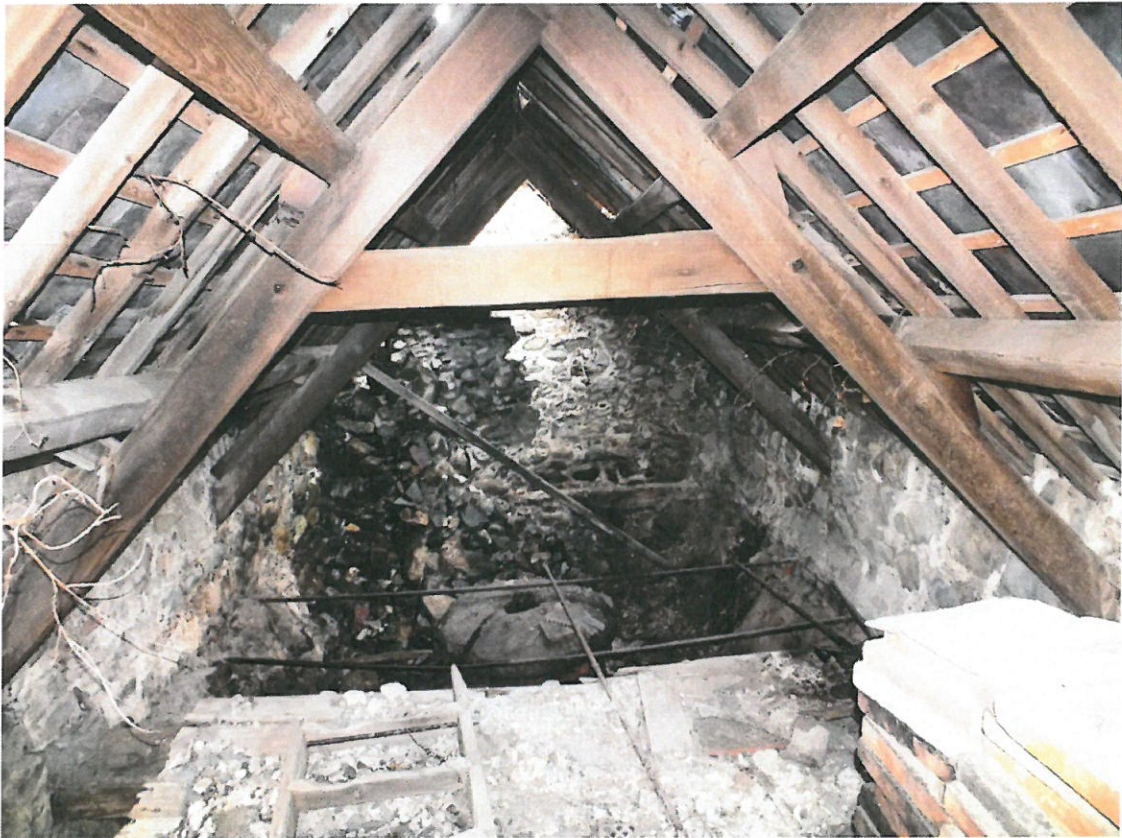
49 Area C – Roof Construction
