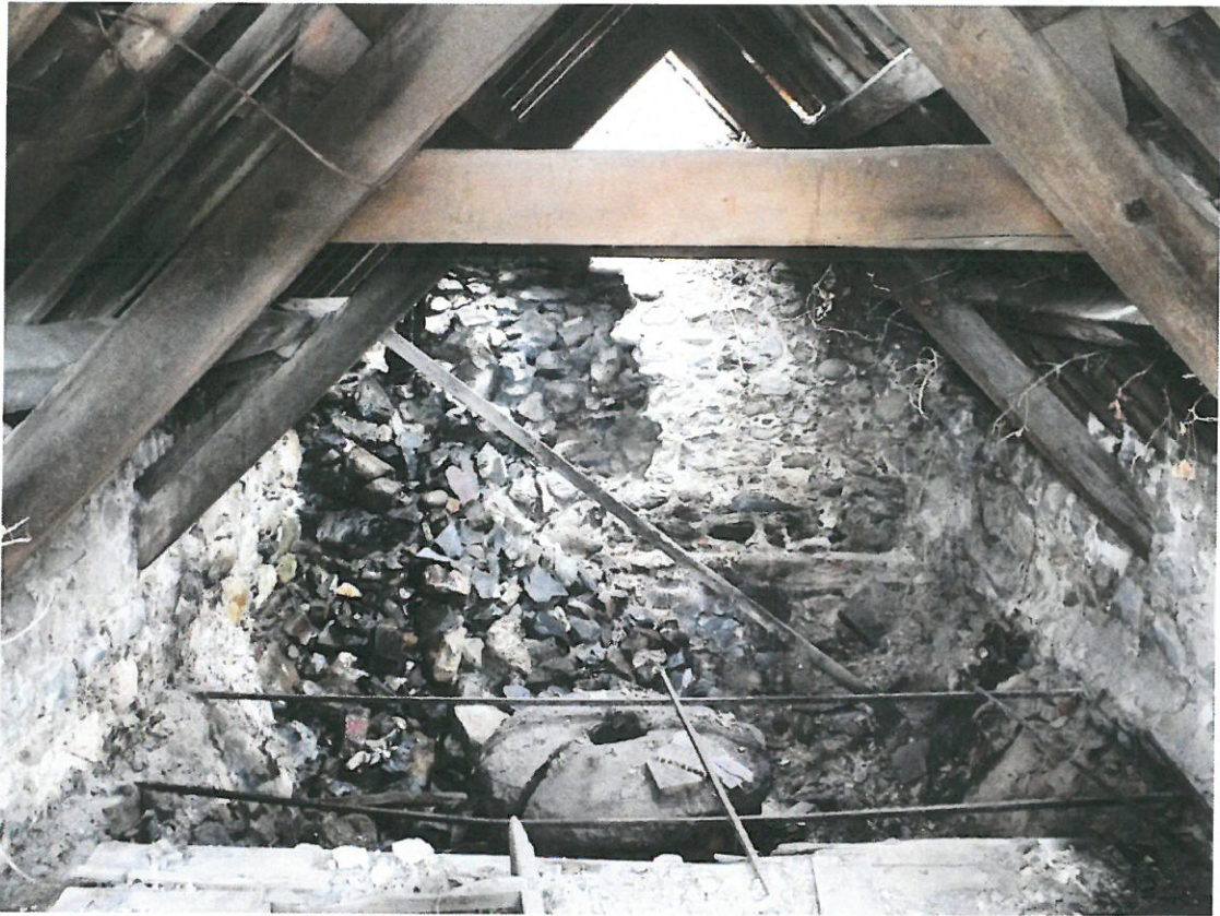
Area C – North-East Wall Collapse
