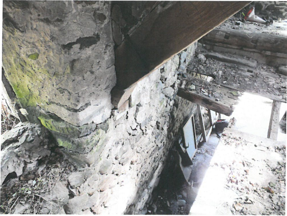
Area A – Truss 2 – Bottom Tie Cut Away
