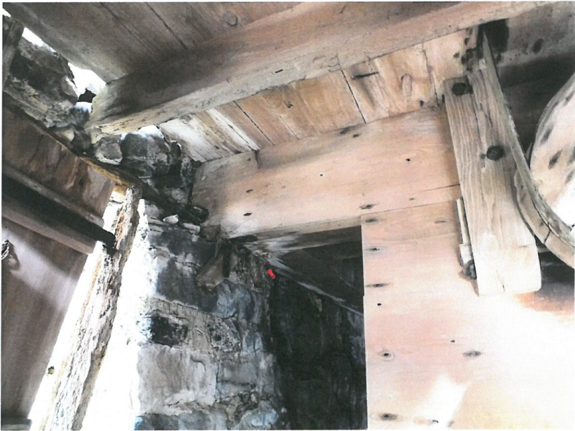
Area B – Beam to Machinery Frame into North-West wall
