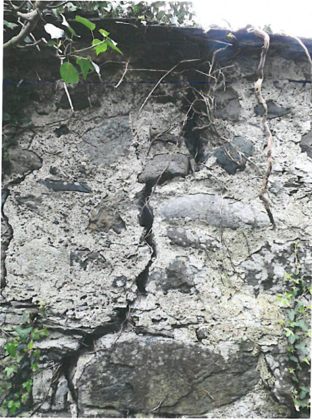
North-East Elevation – Area A – Vertical Crack
