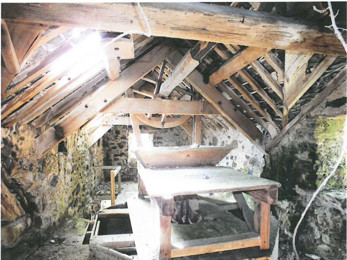
42 Area B – Truss 3
