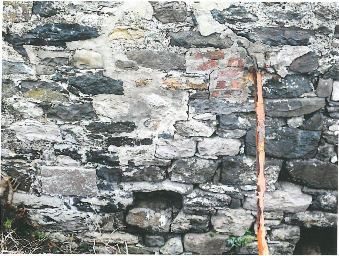
North-West elevation – Area A – Vertical Cracking
