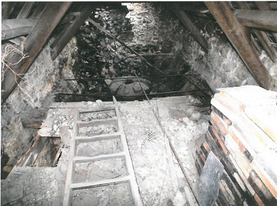
50 Area C – First Floor
