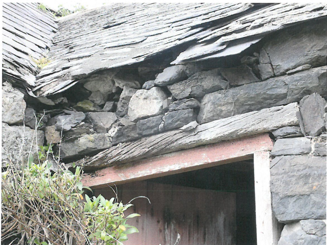
South-East Elevation – Stable – Fragmented Stone
