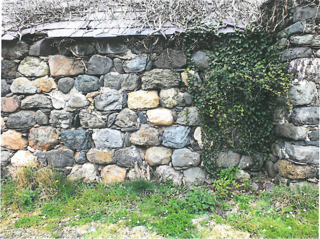
5 South-East Elevation – Area C
