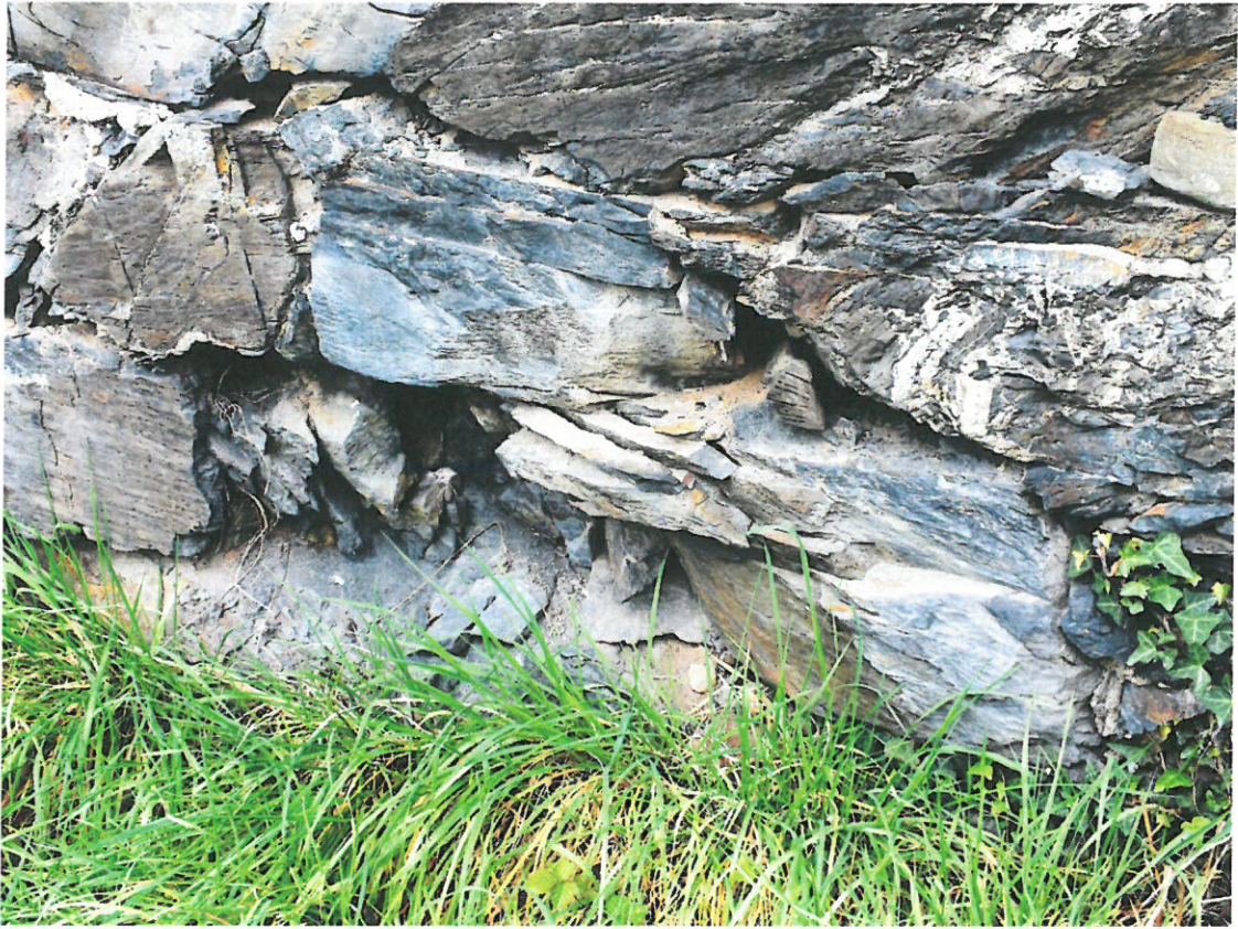
South-East Elevation – Stable – Fragmented Stone
