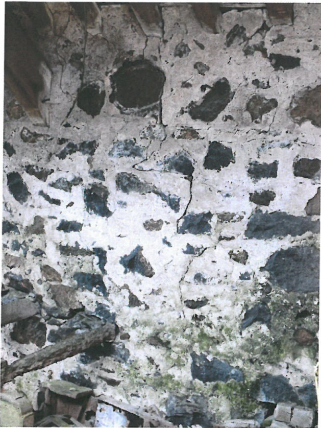
Area B – Vertical Crack in North-West Wall
