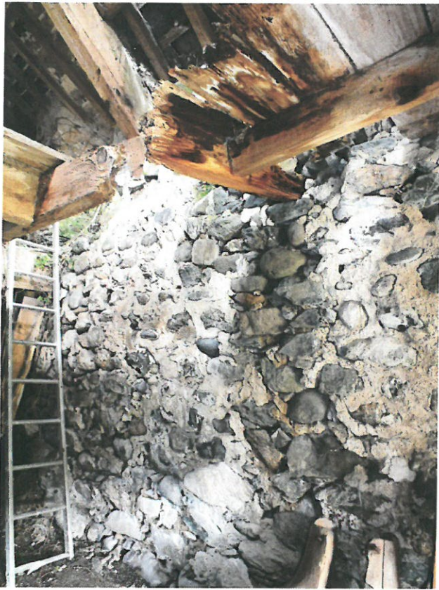
27 Area A – North-East Wall
