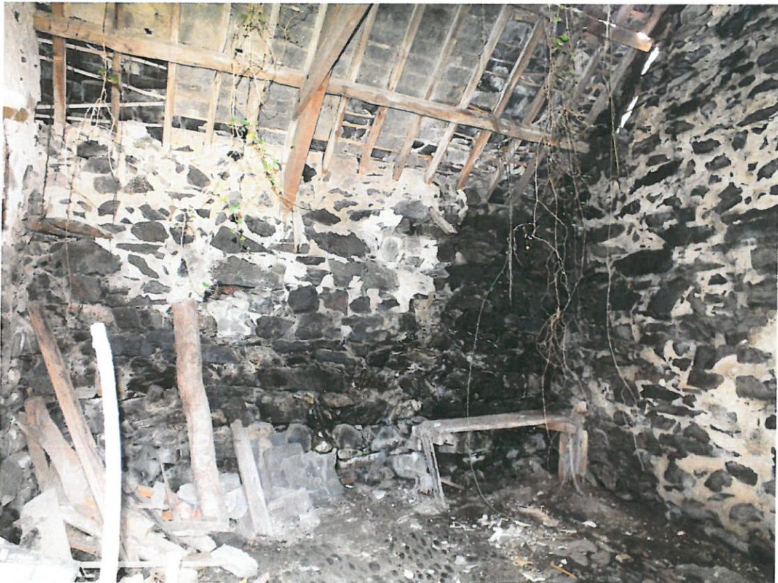
Area C – North-East Wall Collapse
