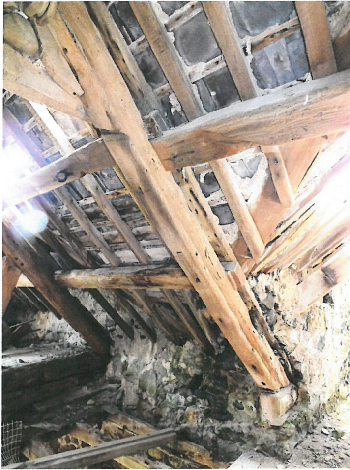
33 Area A – Truss 2
