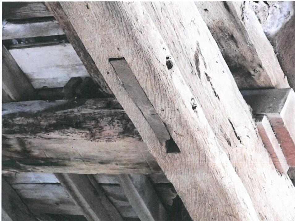
34 Area A – Truss 2 – Collar Removed
