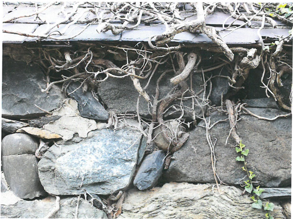
4 South-East Elevation – Area C
