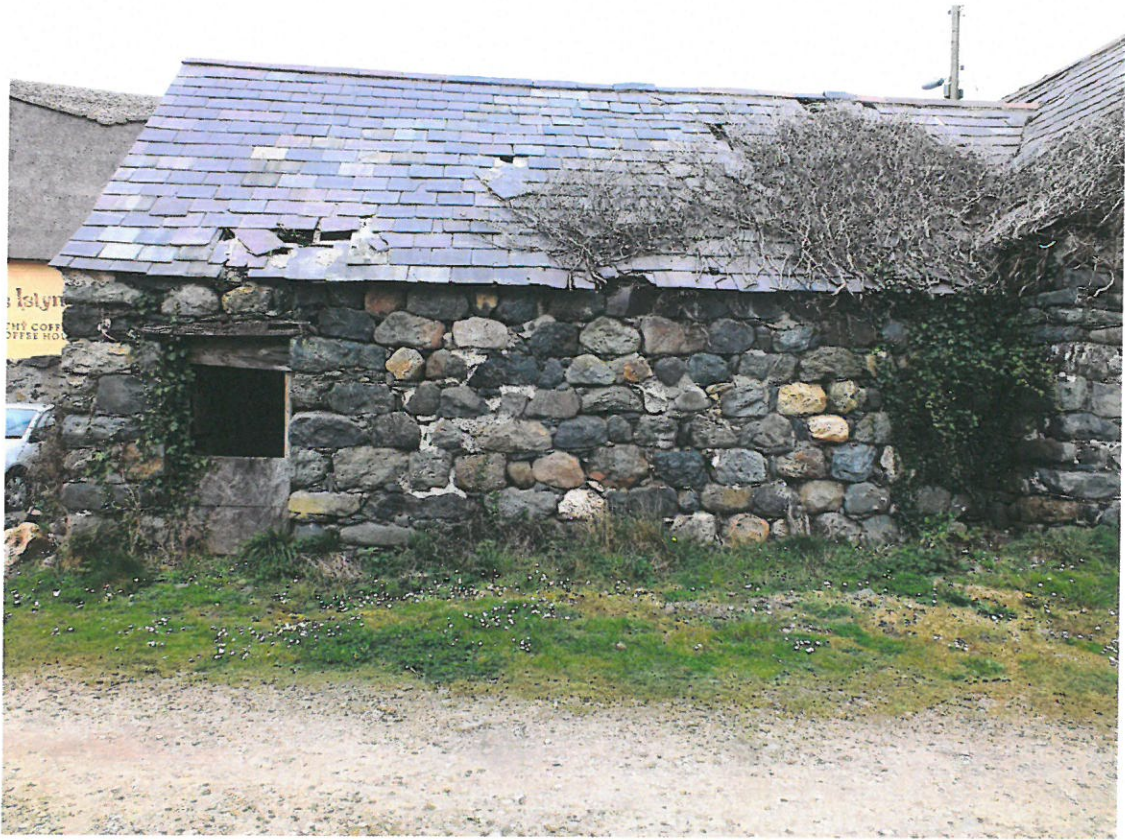
3 South-East Elevation – Area C
