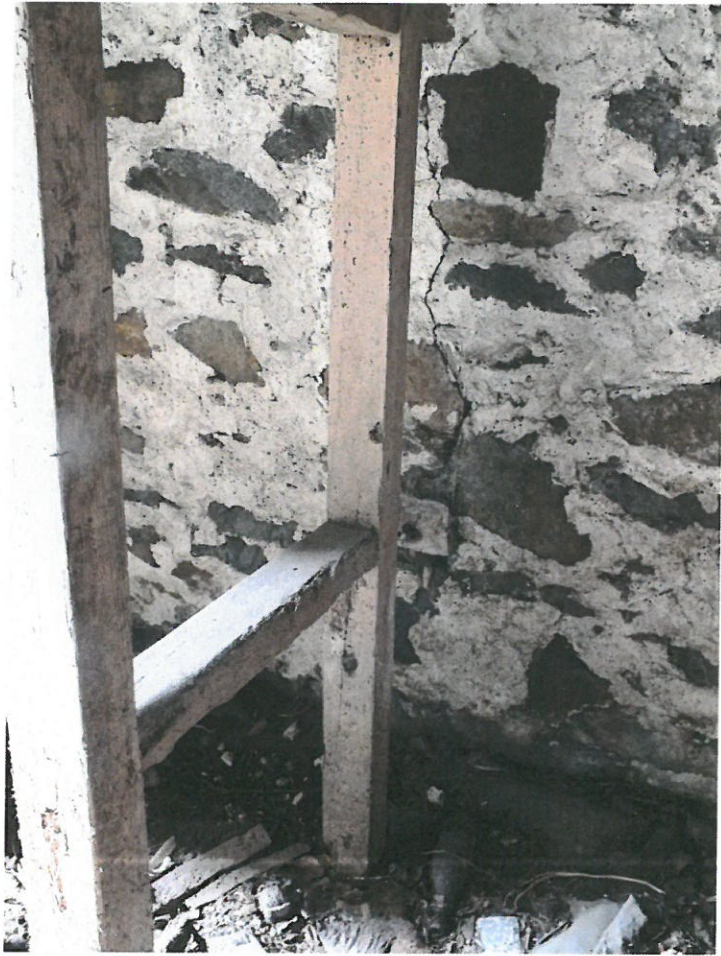
Area B – Vertical Crack in North-West Wall
