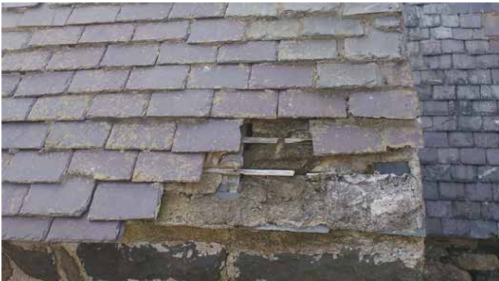
Figure 4. Area 1. Talley slating and mortar bedding of the eaves slates.
