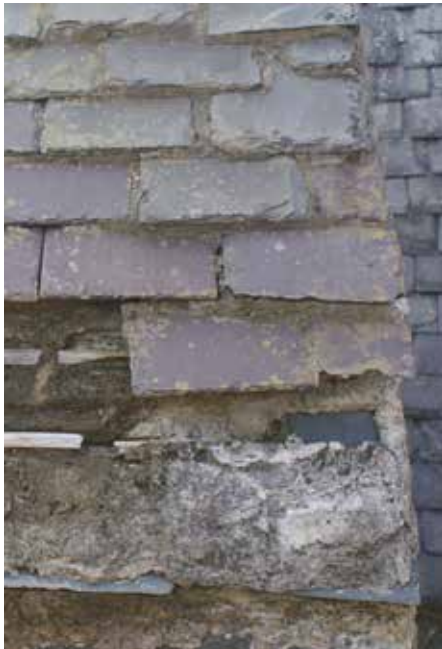
Figure 12. The half bond at the tally slate verges has been closed with various width rather than exactly half slates or slate-and-a-half width slates
