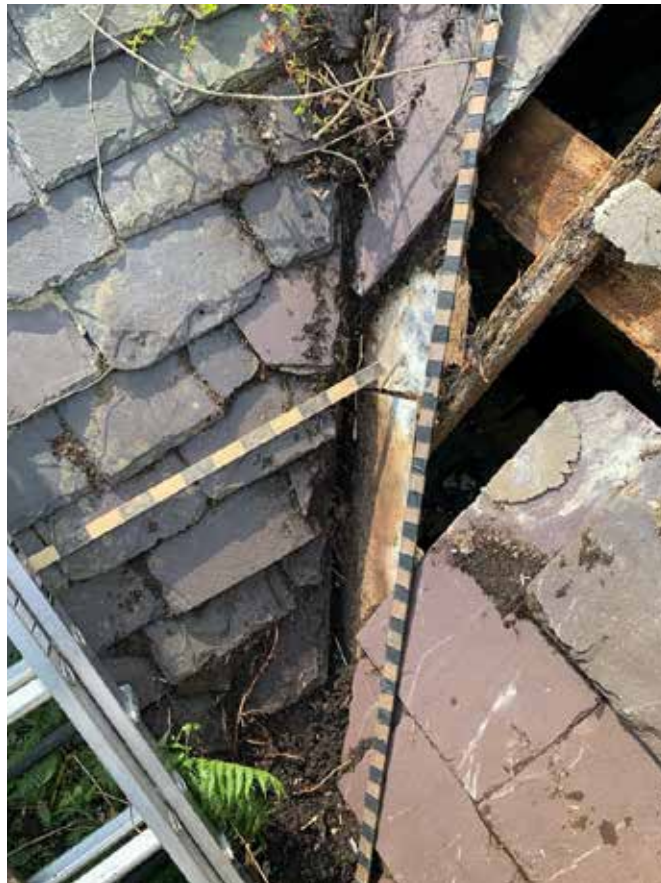
Figure 8. The (split) metal lined valley between areas 4 and 5.
