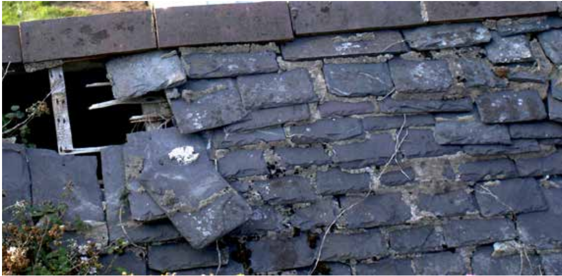
Figure 7. Area 4. Mortar grouting applied to secure failing slating.
