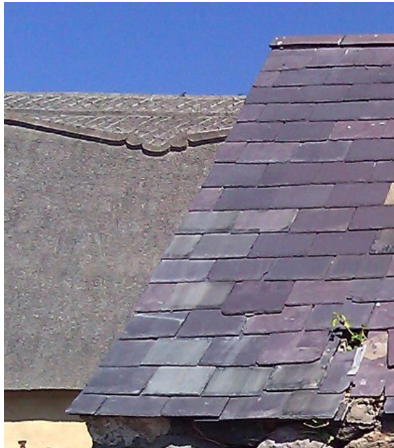
Figure 12. The half bond at the tally slate verges has been closed with various width rather than exactly half slates or slate-and-a-half width slates
