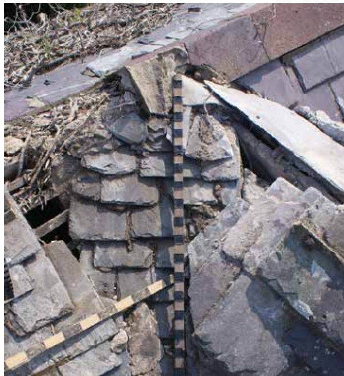
Figure 9. The Welsh valley showing the slating from areas 1 and 2 overlying the valley slates.
