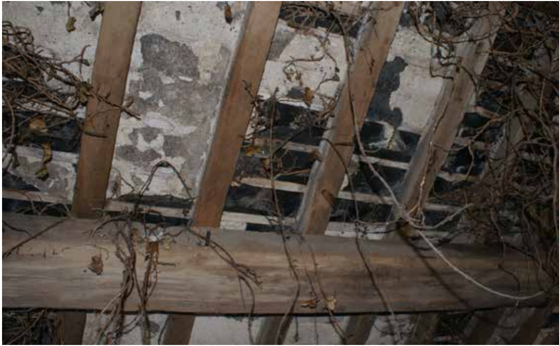
Figure 5. Area 3 Top hung slating on riven laths and torching.
