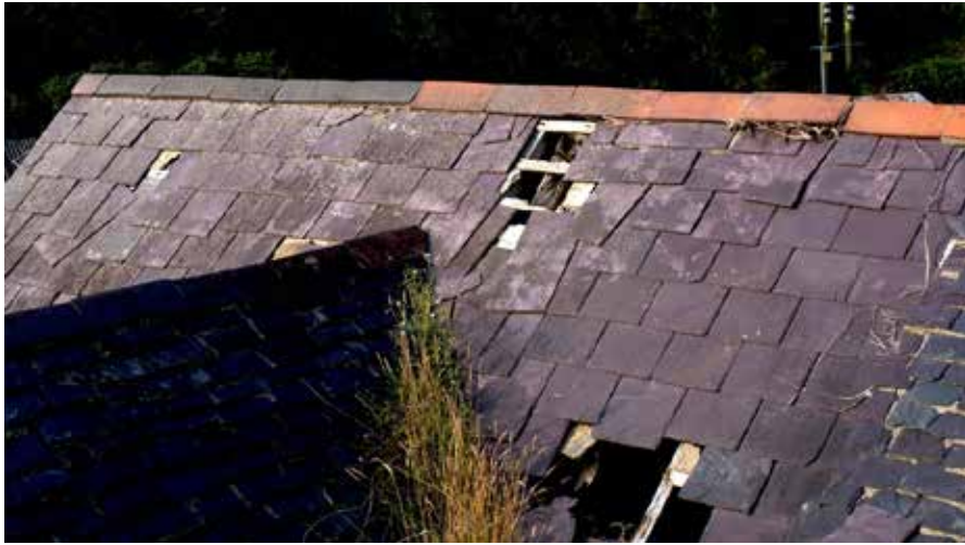
Figure 11. Area 5. Blue brindle and red plain ridge tiles.
