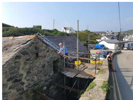
Recording and assessment of the traditional Welsh valley taking place.
