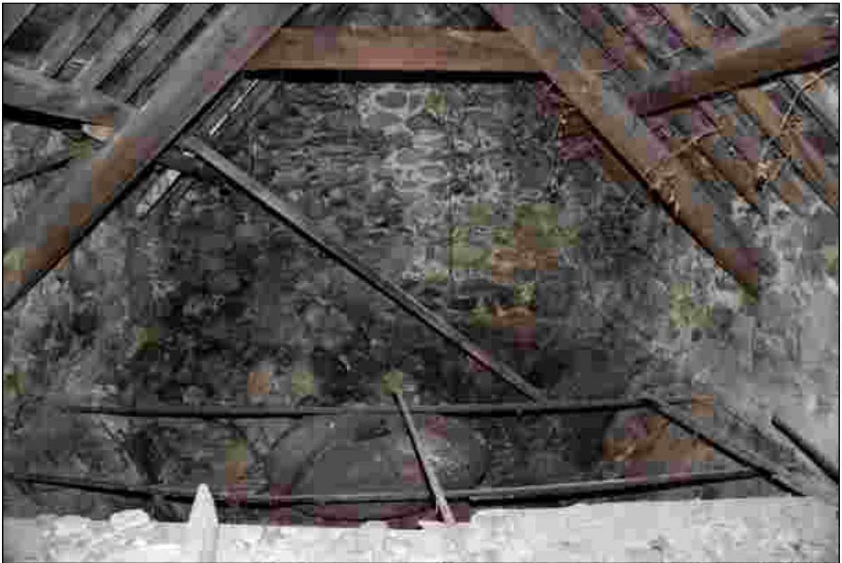
Plate 44: First floor of the corn dryer looking north east.
