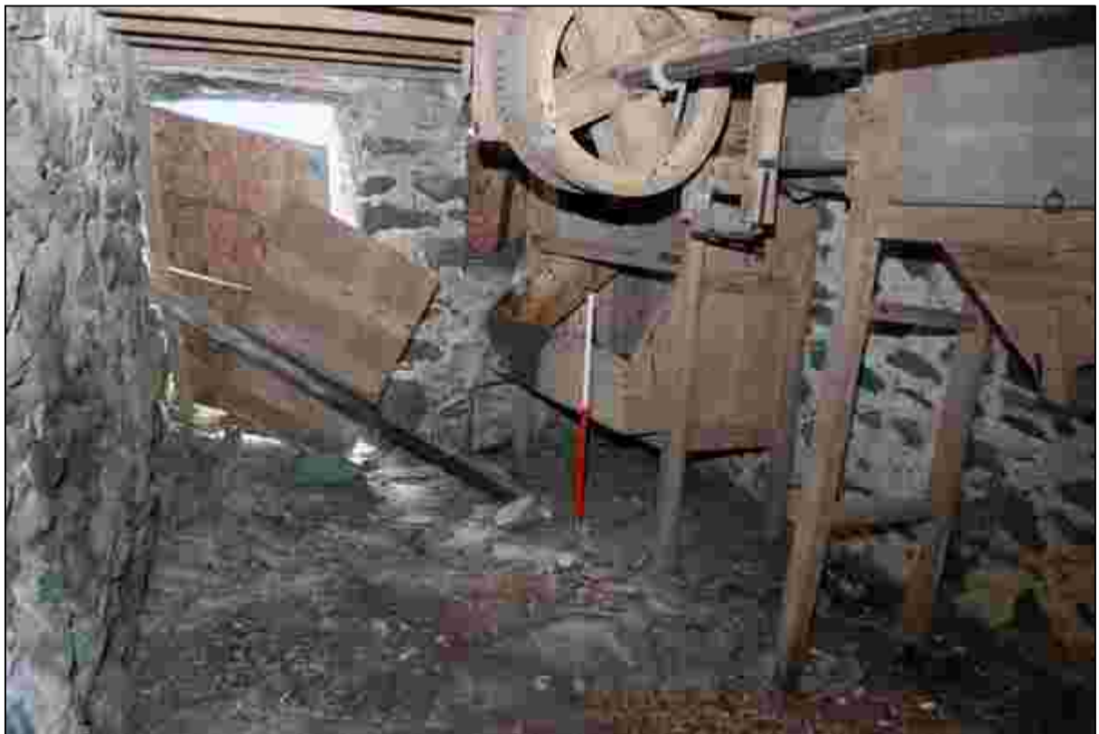
Plate 54: Ground floor of the “Dresser Range”, looking south west
