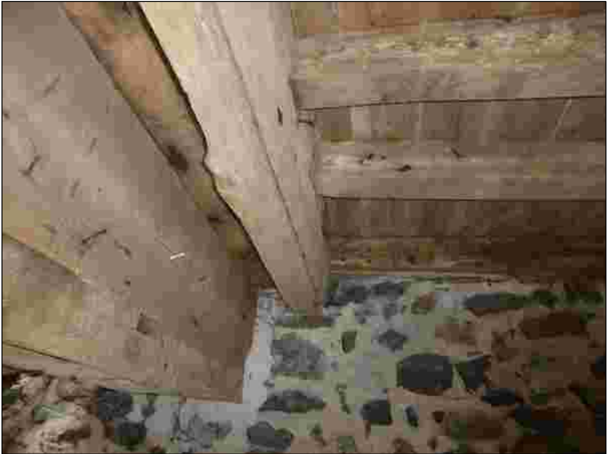
Plate 17: Ceiling joist in the mill range
