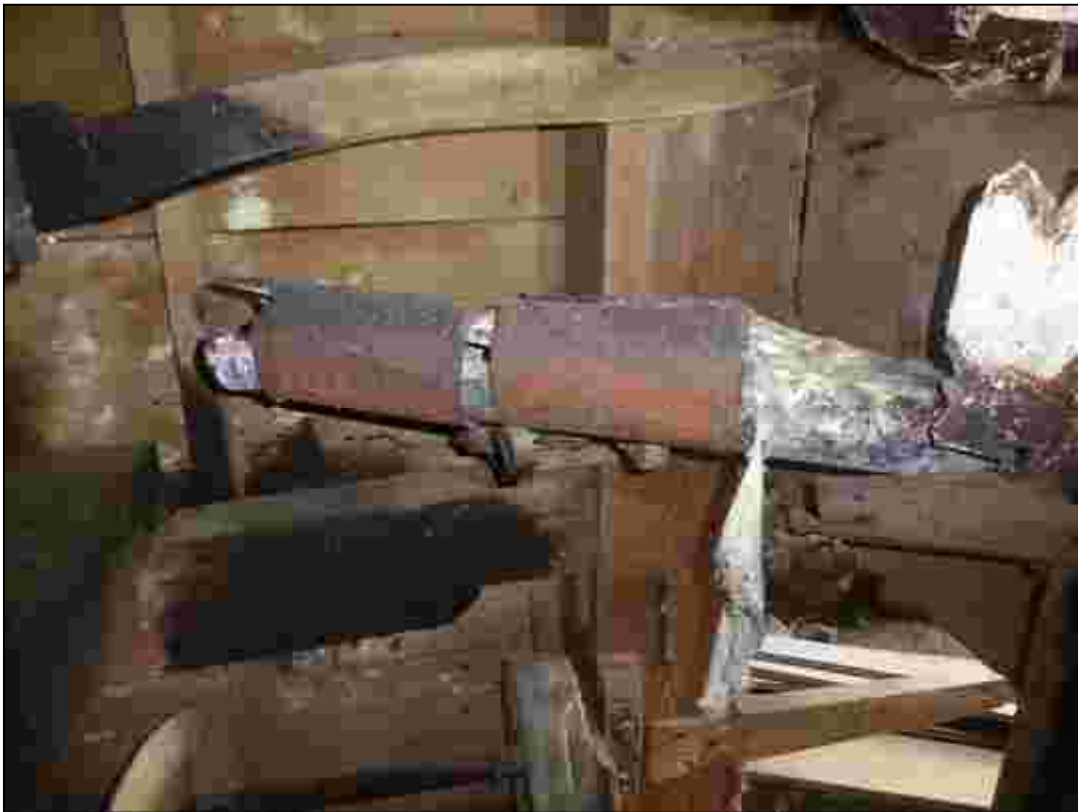
Plate 82: The remains of the chute from the western stones
