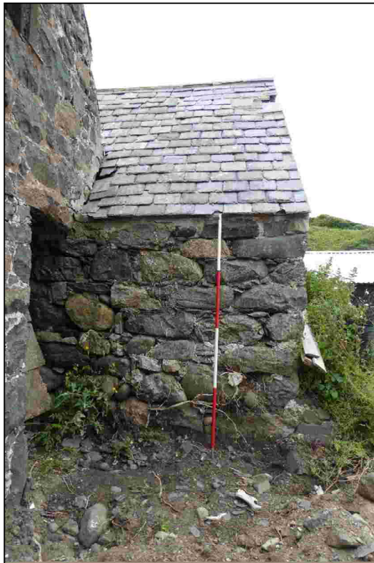
Plate 34: Northern elevation of the corn dryer
