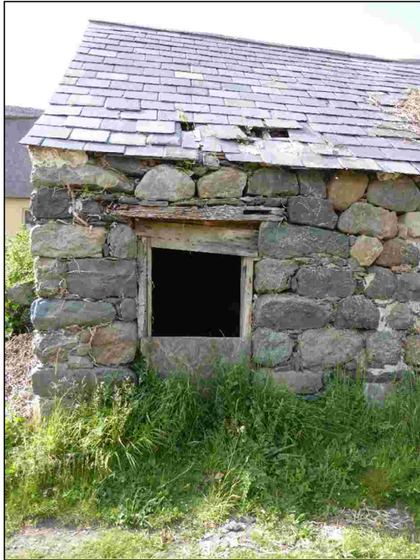
Plate 31: Ground floor entrance to the corn dryer
