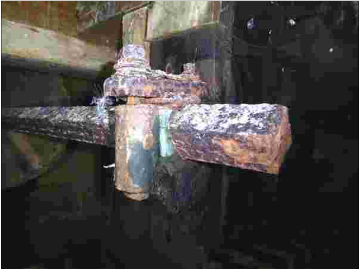
Plate 83: The bearing at the eastern end of the lower lay shaft
