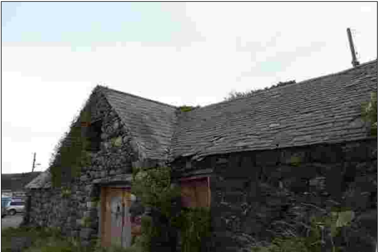
Plate 8: The roof of the mill range
