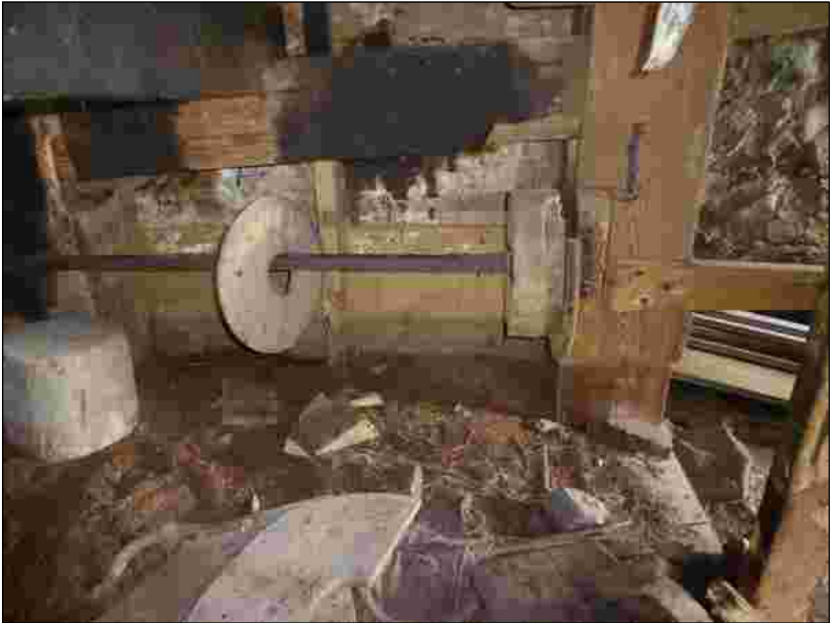
Plate 87: Shaft at the foot of the Hurst Frame
