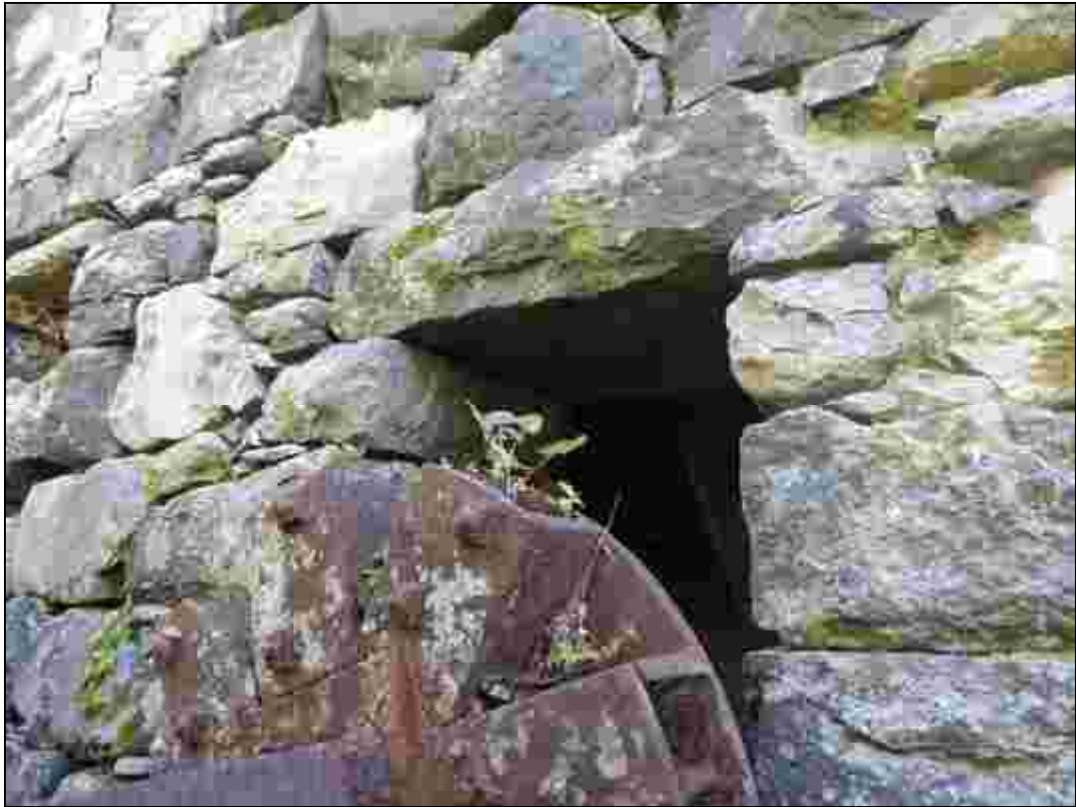
Plate 11: The opening for the water wheel axle
