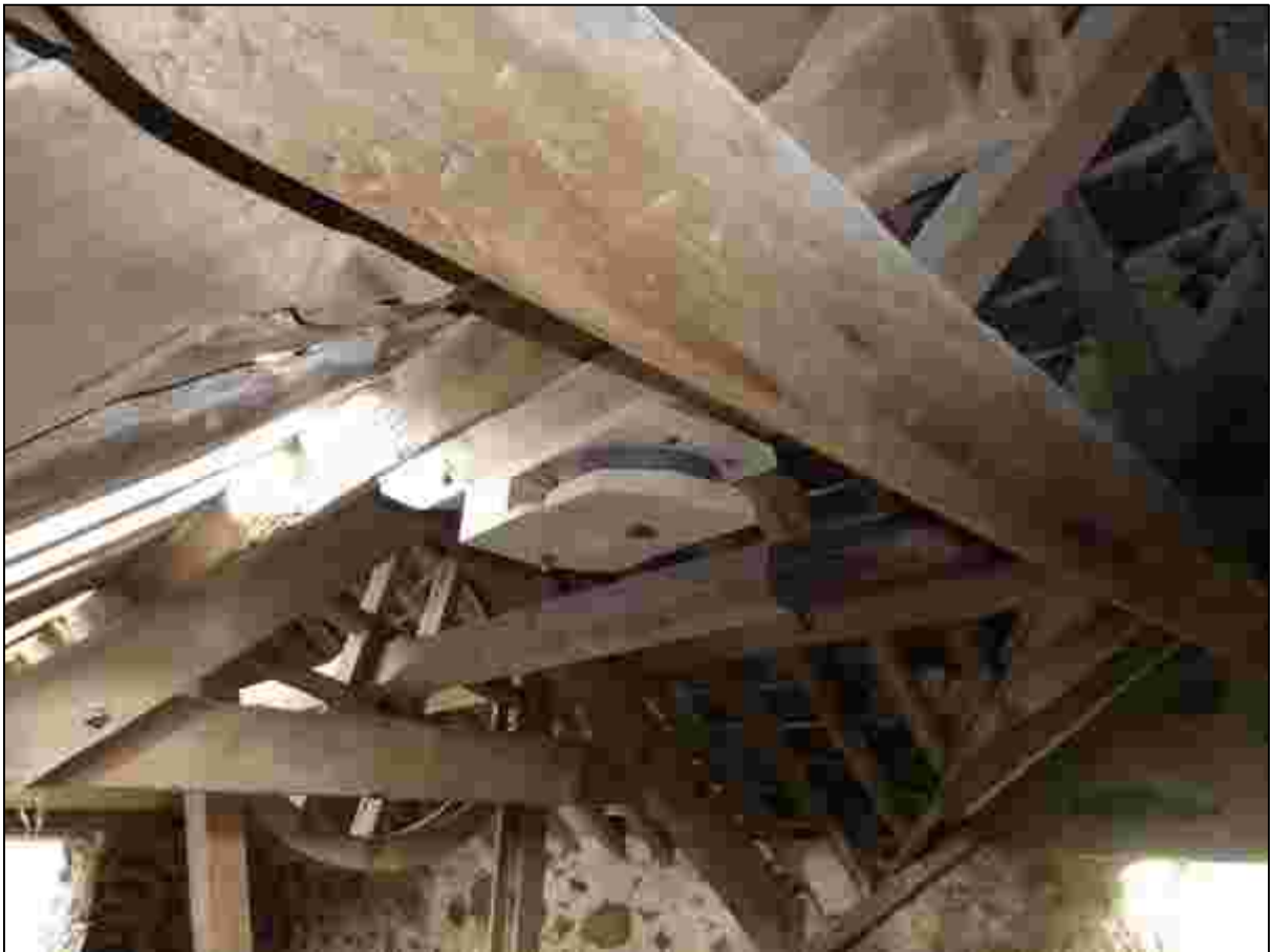
Plate 100: Pulley wheel, part of the sack hoist mechanism
