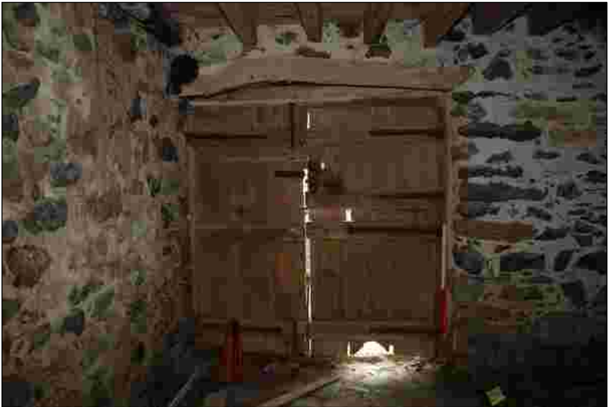
Plate 14: Inside of the doors to the mill range
