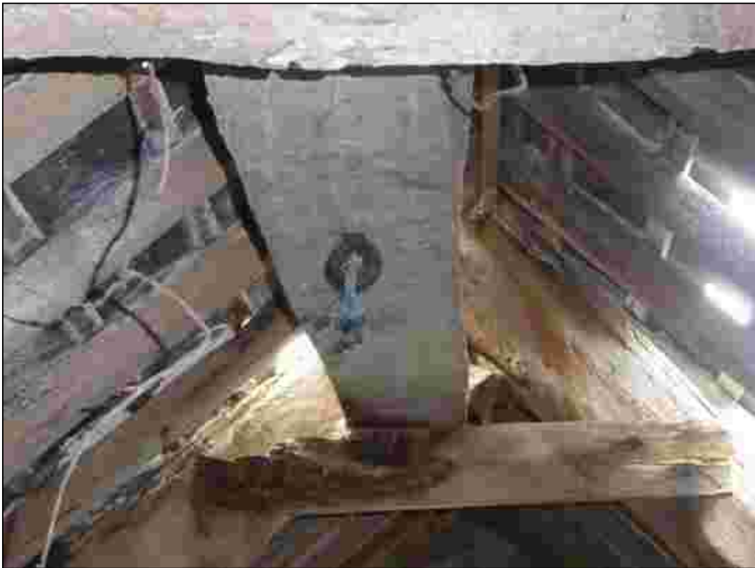
Plate 26: Iron ring above the hatch in the mill range.
