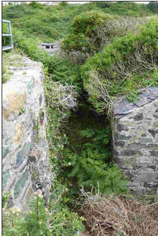
Plate 6: Shallow buttress on the pond retaining wall
