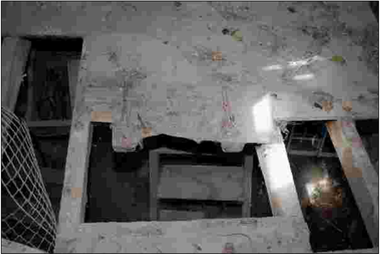
Plate 23: Remains of the hatch in the mill range
