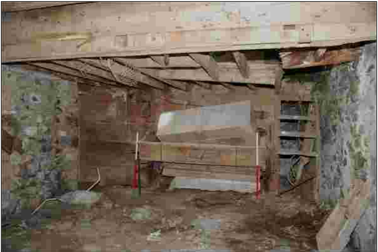
Plate 20: The Hurst Frame and trough in the mill range
