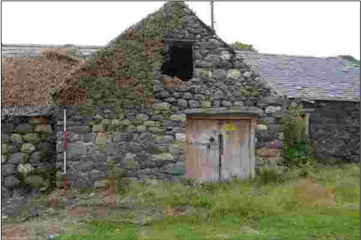
Plate 7: The south eastern gable of the mill range
