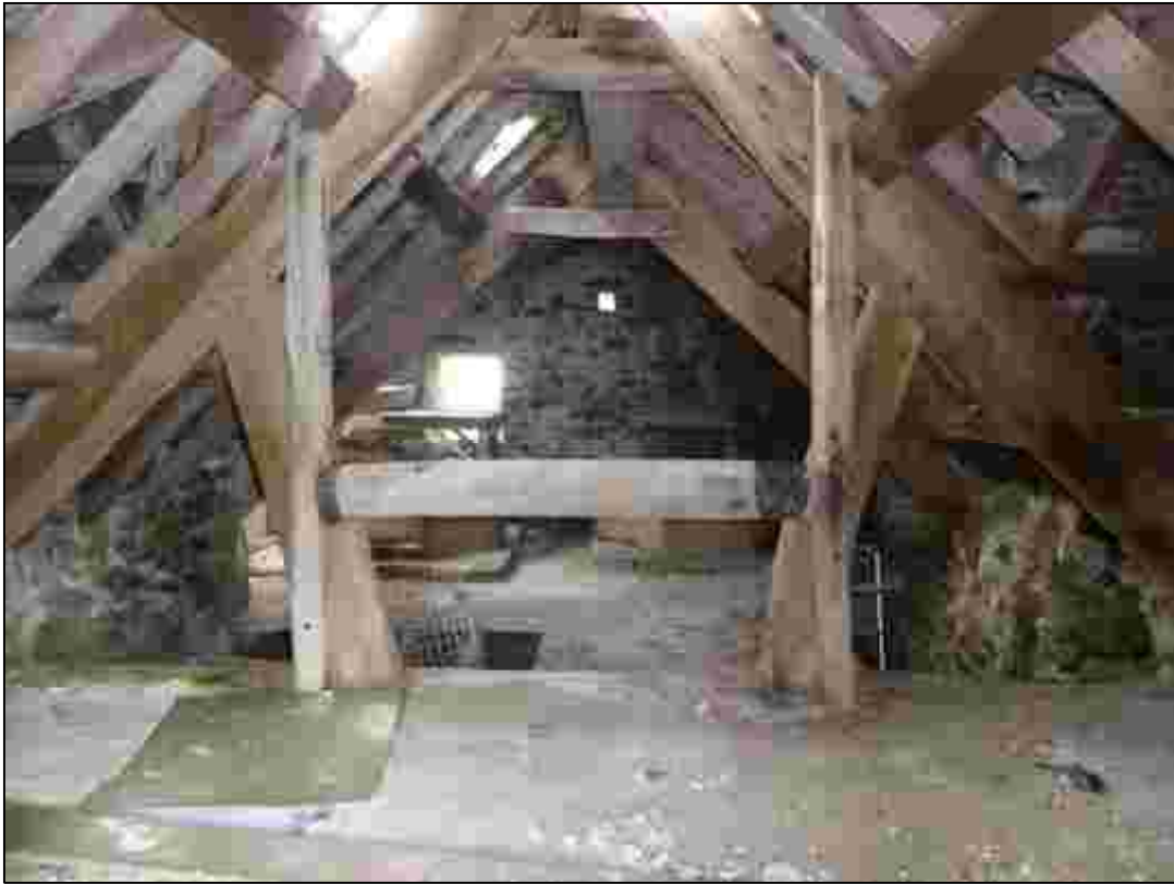
Plate 25: The windlass attached to Truss 1
