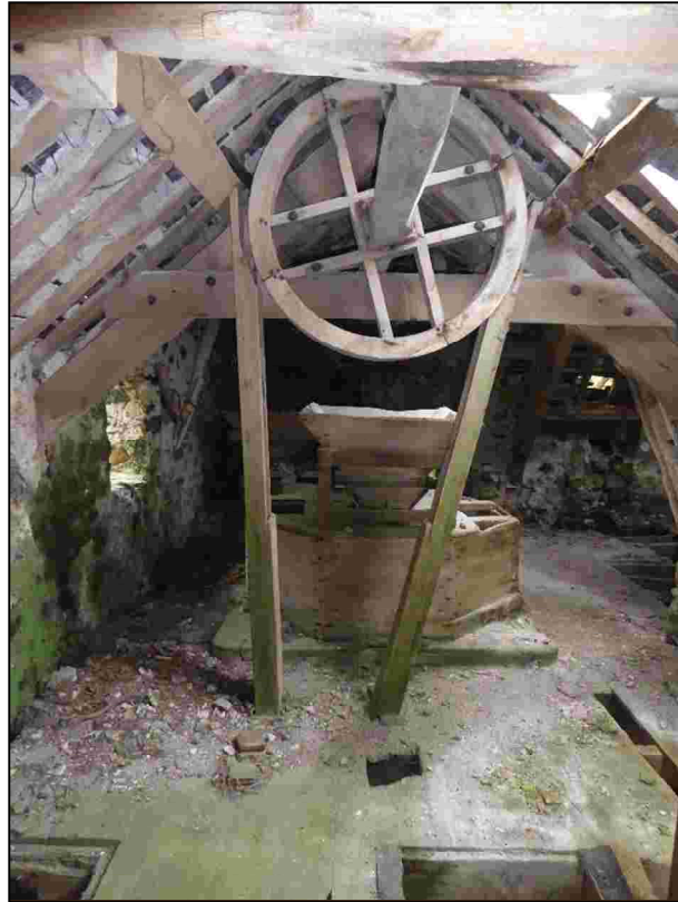
Plate 97: The upper pulley wheel.
