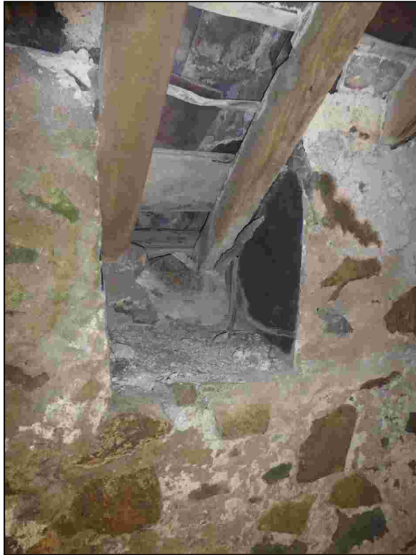
Plate 59: Detail of the slate lined niche
