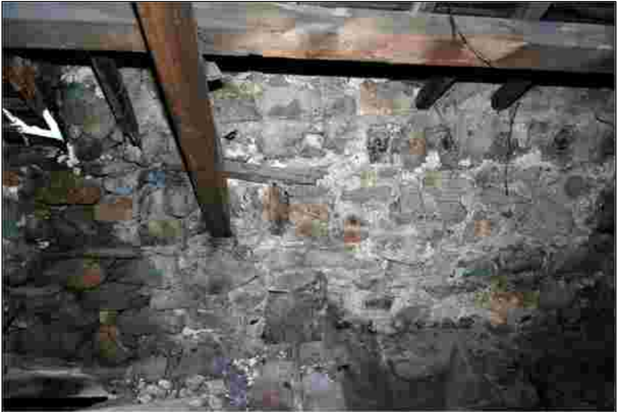
Plate 47: Sawn off principle rafter
