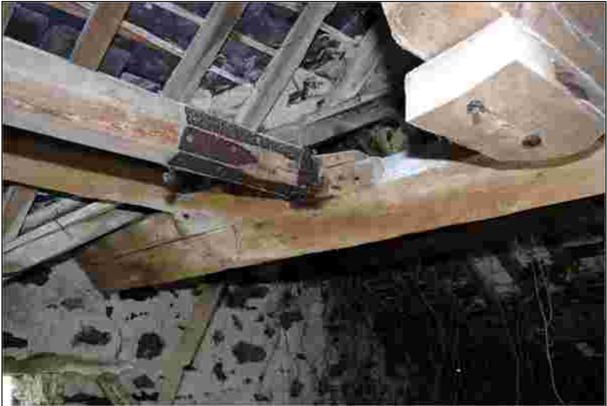
Plate 99: The reinforced section of the upper lay shaft
