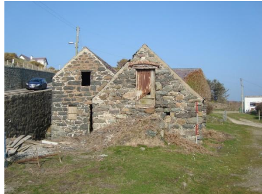
Melin Aberdaron viewed from the west, showing (a) to the right, the wing containing the kiln and a first-floor room accessed by steps, and (e), which contains the dresser. These two parts appear to belong to different periods of construction.
