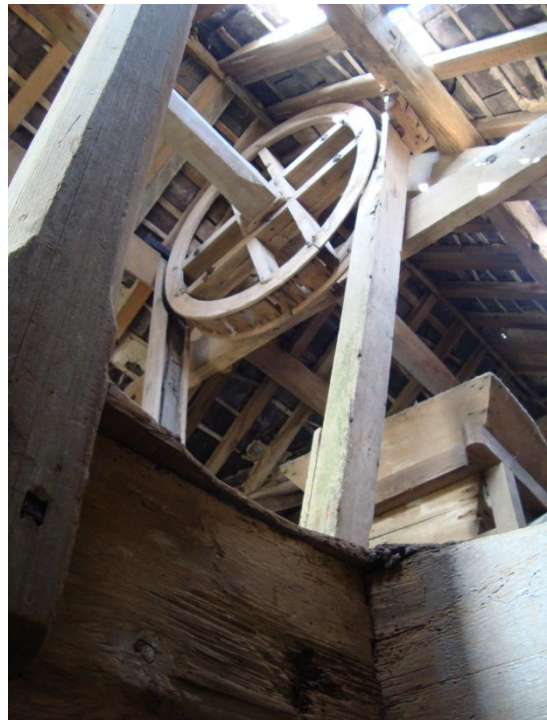
The sack-hoist, showing the clasp-arm belt wheel and the wooden guards for the belt-drive.
