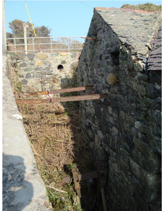
The wheelpit from the west
