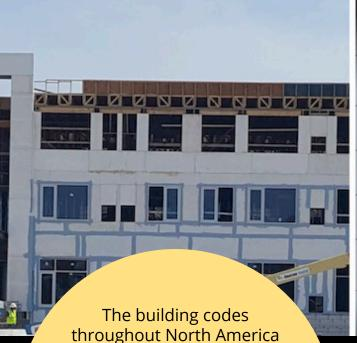
throughout North America are demanding better energy performance. The use of continuous external insulation is now a requirement to meet the codes in virtually all steel-frame buildings and many wood-frame structures.
