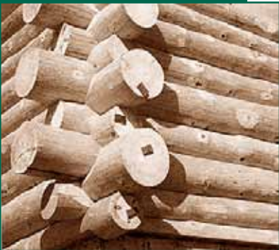
Figure 5-7: Log wall construction
