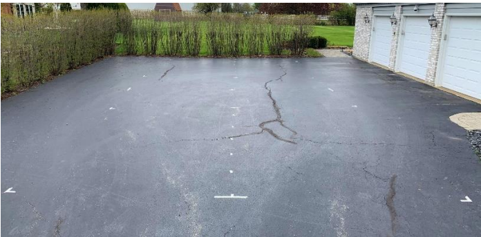
Fred Phillips marked where lines will be painted in drive.
