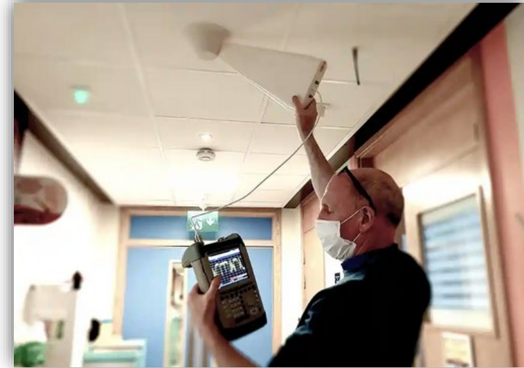
End-to-End WiFi Distributed Antennae And Structured Cabling Installation And Service
