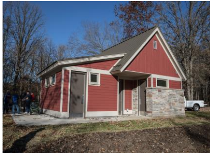
Toilet/shower bldg. constructed 2017
