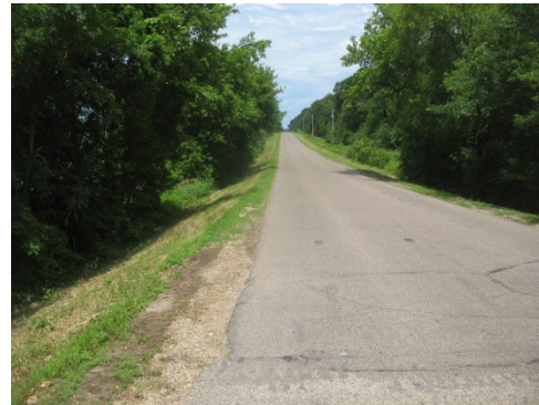
Existing Conditions, Anderson Scout Camp Trail
