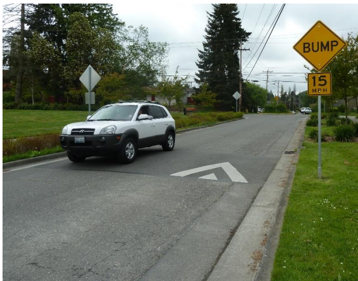
Traffic calming aims to slow the speeds of motorists through a variety of treatments, such as the speed hump shown above.
