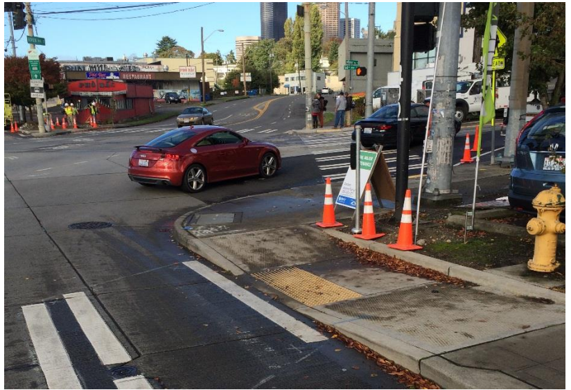
Curb ramps must include truncated domes. Sedimentation and snow accumulation are challenges.
