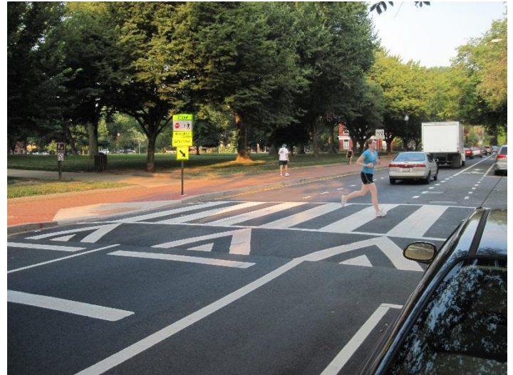
Raised crosswalks have traffic-calming effects. This crosswalk crosses two travel lanes, a bike lane, and a parking lane.
