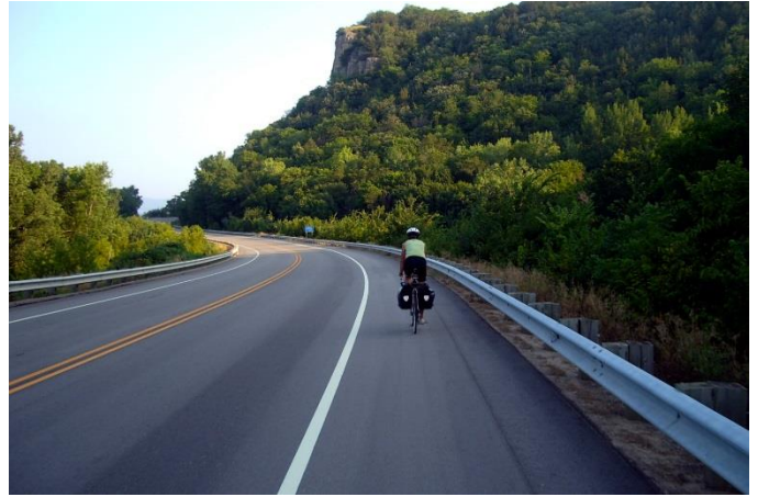
Paved shoulders reduce run-off-road crashes, improve roadway maintenance, and can provide space for bicyclists
