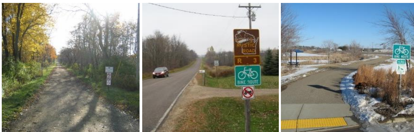
Examples of the results of previous planning efforts in St. Croix County. The Wildwood Trail (left), a signed bike route (center), and Hatfield Lake Trail in New Richmond (right).
