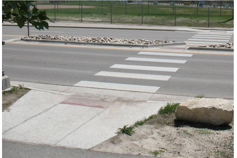
Crossing islands with offset openings encourage pedestrians to face oncoming traffic before crossing the opposite side of the street.
