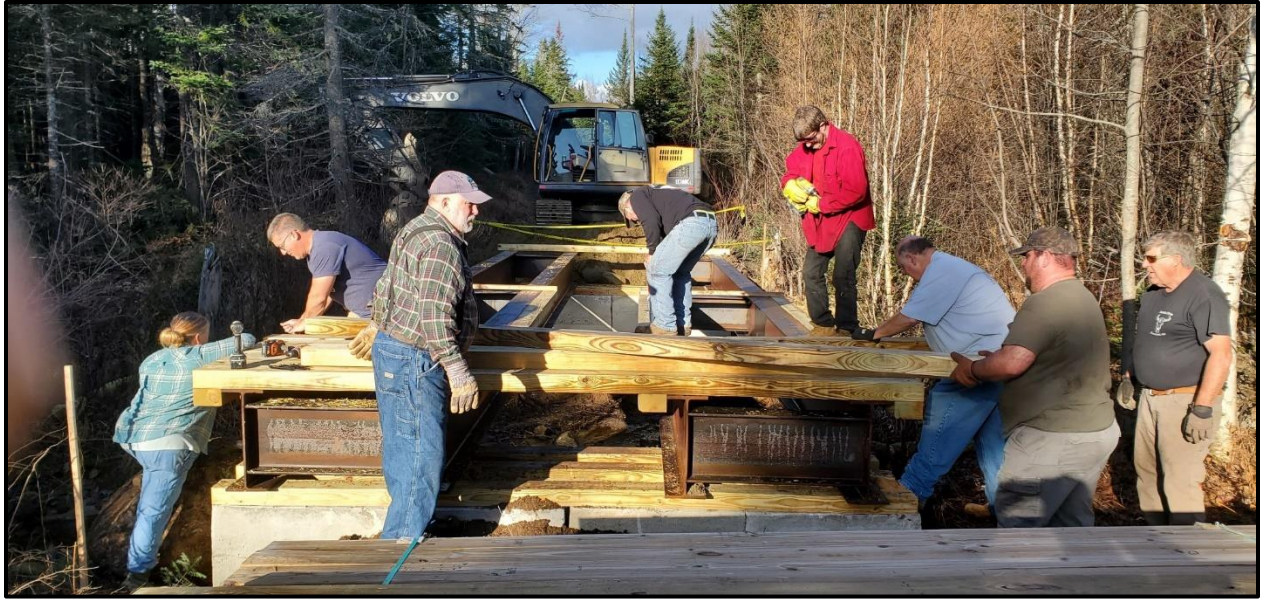
The crew just finished installing the stringers next to the steel beams and are just starting to install decking.
