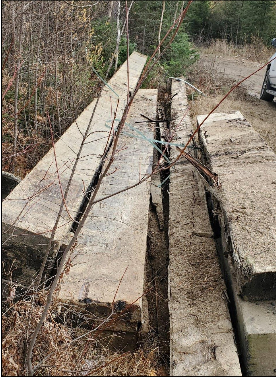
Two of the three wood beams from the old bridge are being recycled by the Presidential Range Riders snowmobile club to build a temporary bridge over a large washout in Gorham. The third beam was broken in half and could not be used.
