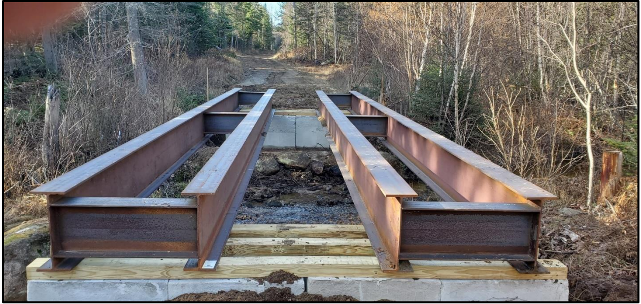
Steel beams set on top of cement abutment blocks ready for decking.
