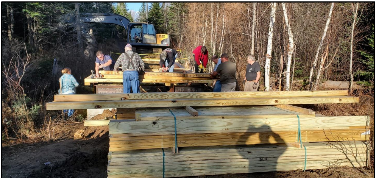
Some of the crew transferred the heavy deck boards from the lumber pile to the bridge while other crew members used cordless drills to fasten the deck boards to the stringers using Timberlok screws.
