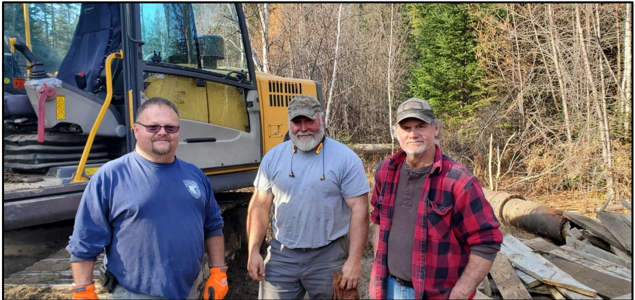
The Friday crew responsible for dismantling the old bridge and getting the abutments and steel in place for the new bridge. (Left) Clint Savage District 1 Supervisor from the NH Bureau of Trails, (Middle) Don Doucette excavator operator from Romik Developers and (Right) Kevin Wyman from the NH Bureau of Trails.
