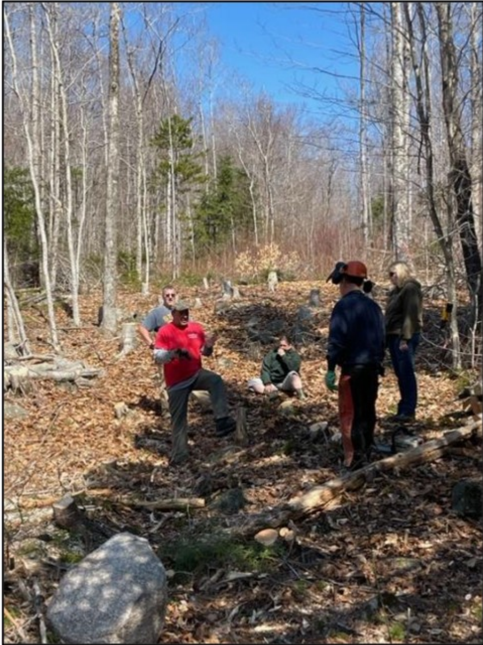
The crew takes a break after clearing several dozen trees.
