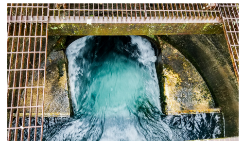
The weirs on the dam are unaffected by the increased flows
