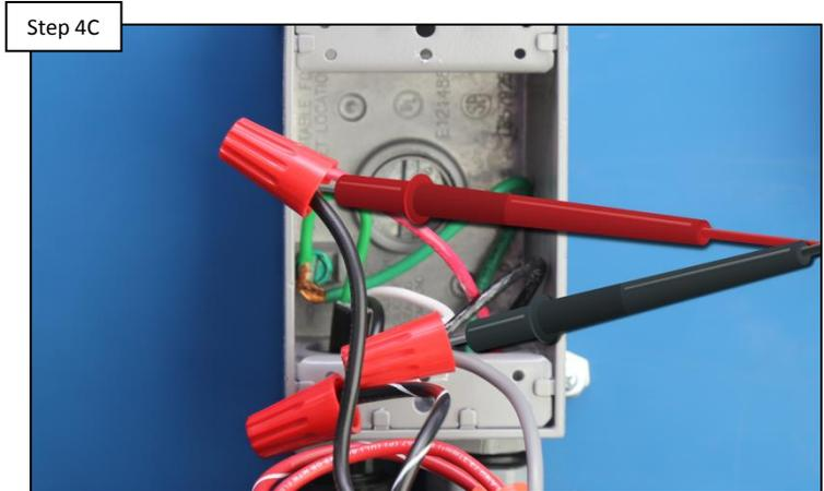
Verify line power to the Smart Relay between the grey & black (120vAC) or black & red/grey (240vAC). IF no/low voltage, correct at power source. IF correct, replace the Smart Relay ([HLX485RELAY](#)).
