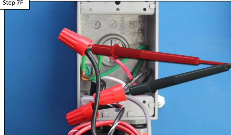
Test the Smart Relay's input power for 102-138vAC. IF power is correct replace the Smart Relay (**HLX485RELAY**). IF no/low voltage, resolve at breaker.
