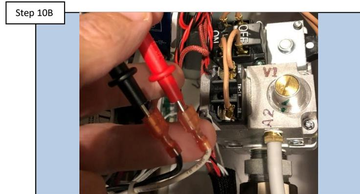
Press the mode button to toggle the heater and call for heat. IF 24VAC is not present at gas valve AND manifold pressure is present, gas valve is defective and needs to be replaced. Otherwise, replace the ICB ([pg. 25](#)).
