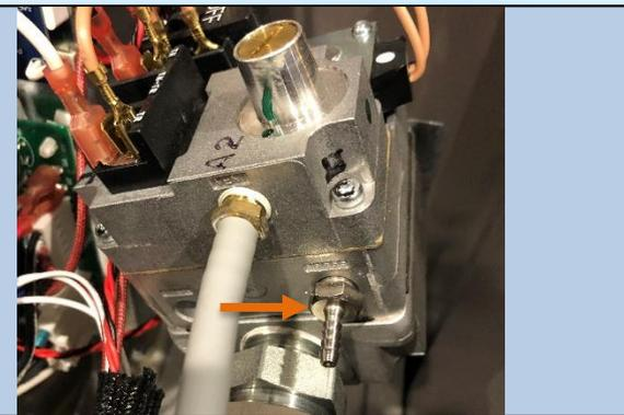
Install barbed fitting from manometer in the pressure port of the gas valve..
