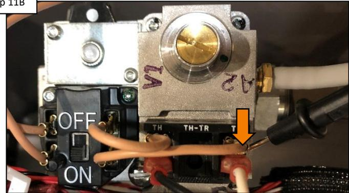
With filter pump running, take one lead from your multi-meter and place it on the terminal with the white wire on the gas valve, then Go To Step 11C.
