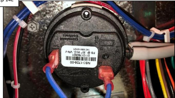
Verify diff. pressure switch is open when blower is off, turn heater on and check to see if dps switch closes. IF NOT, replace switch. IF problem persists, contact Technical Support at (908) 355-7995.
