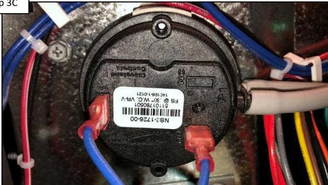
With power off, inspect the diff. pressure switch wiring for damage. IF damaged, replace the wire harness (pg. 25). IF OK, go to step 3D.
