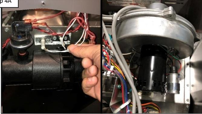
Inspect the Ignitor & Blower wiring. Verify insulation is not damaged. IF wires are damaged, replace the damaged part (pg. 25). IF OK, go to 4B.
