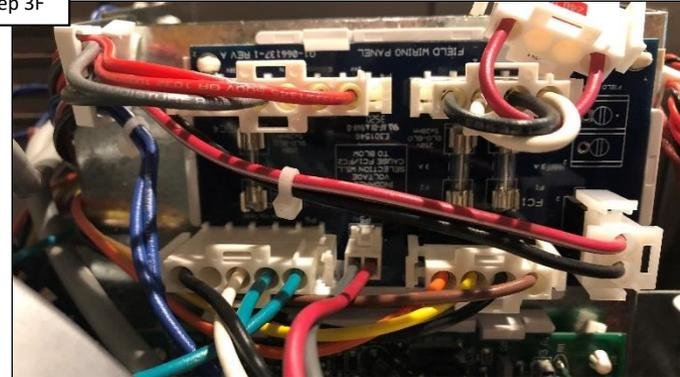
Inspect ICB wiring. IF wiring is damaged, replace the wire harness with a new wire harness kit (pg. 25). IF OK and the problem still exists, replace the ICB (pg. 25)
