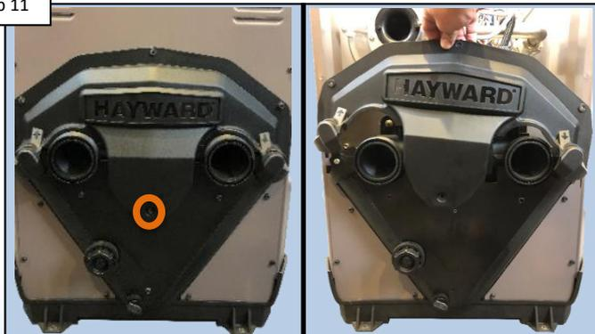
Remove the center screw (left pic.) from the header controls cover. Remove controls cover (right pic) by lifting up on the cover.
