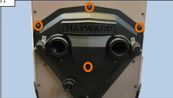
Turn power off, remove the 4 screws from the header controls cover and remove the panel.
