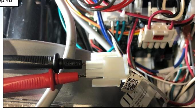
Disconnect ignitor from ICB & measure resistance of ignitor. Verify 8-25 ohms between 20°-140°F. IF correct, go to 4C. IF NOT, replace ignitor (pg. 25).
