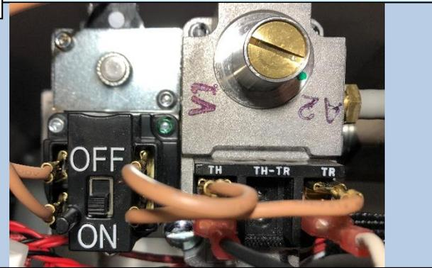
Verify that the gas valve, inside the heater, is in the "ON" position. IF correct, go to step 12C. IF NOT, slide switch to "ON" position.
