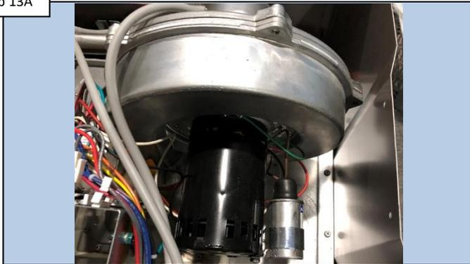
**With the heater off (in “Stand By”), IF the blower continues to run/operate, replace the ICB (pg. 25).
