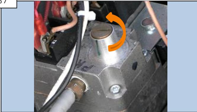
Remove plug from gas valve with a flat head screwdriver. Go to Step 8
