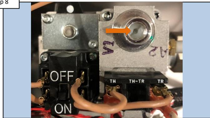
Once removed, increase pressure by rotating screw clockwise, (counter clockwise to reduce pressure).
