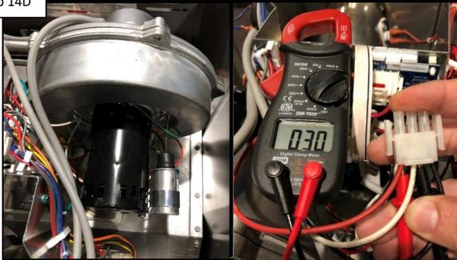
Test the blower for the proper resistance. Measure for 3-5 ohms across red and white terminal wires. IF out-of-range, replace blower (pg. 25). IF OK, go to Step 14F.
