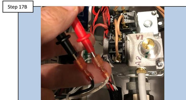
With heater in standby mode, test for 24VAC on the gas valve (black & white wires), IF 24VAC is present, replace gas valve (pg. 25). Otherwise, replace the ICB (pg. 25).
