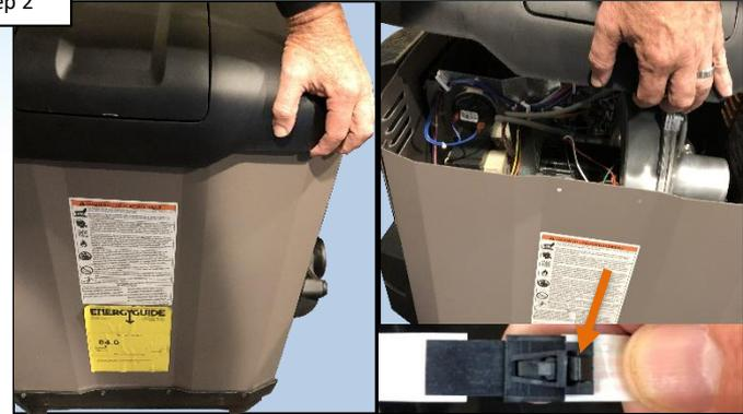
Carefully lift up on the top of the heater cover and disconnect the ribbon cable from the display, then remove cabinet top.
