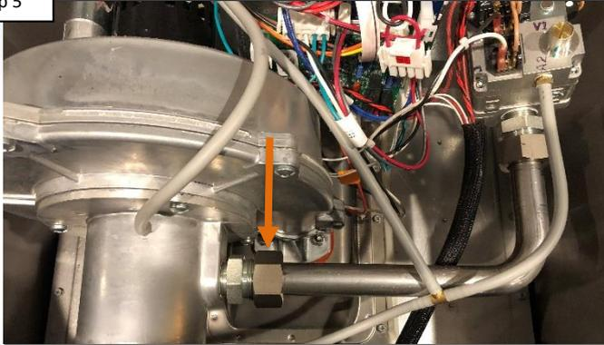
Loosen the flare nut from the gas manifold closest to the blower. Gently pull the manifold out of blower.
