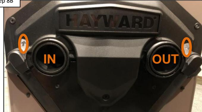
Verify the water inlet & outlet are not reversed; reversing plumbing will cause the “HS” error code. Follow the steps outlined in 8A. IF the thermistor is good, replace the ICB ([pg. 25](#)).
