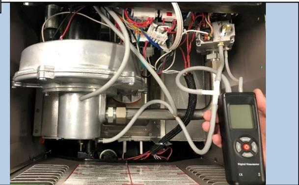
Ensure gas static, load, and manifold pressures are correct (Pg. 13). IF OK, go to Step 12E. IF NOT, go to Step 12F.
