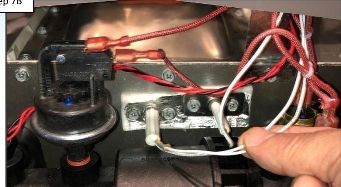
Verify ignitor is securely attached to ICB. If OK, inspect wires for damage. If damaged/worn, replace ignitor (pg. 25) IF OK, go to step 7C.
