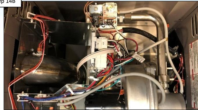
Check blower tubing for damage/loose fit. IF damaged, replace tubing ([pg. 25](#)). IF correct, go to Step 14C.
