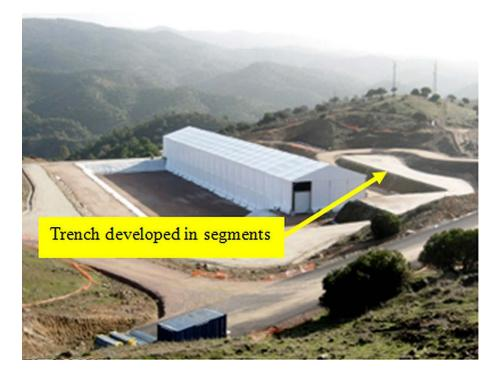
Figure 5-8 Protective Tent Over Active Section [11]
