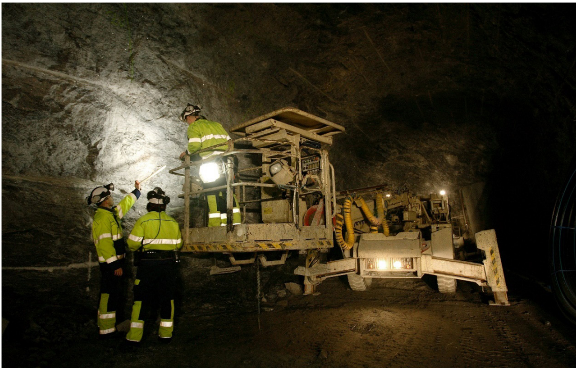
FIG. 18. Construction of the ONKALO underground research facility, Finland (courtesy of Posiva).
