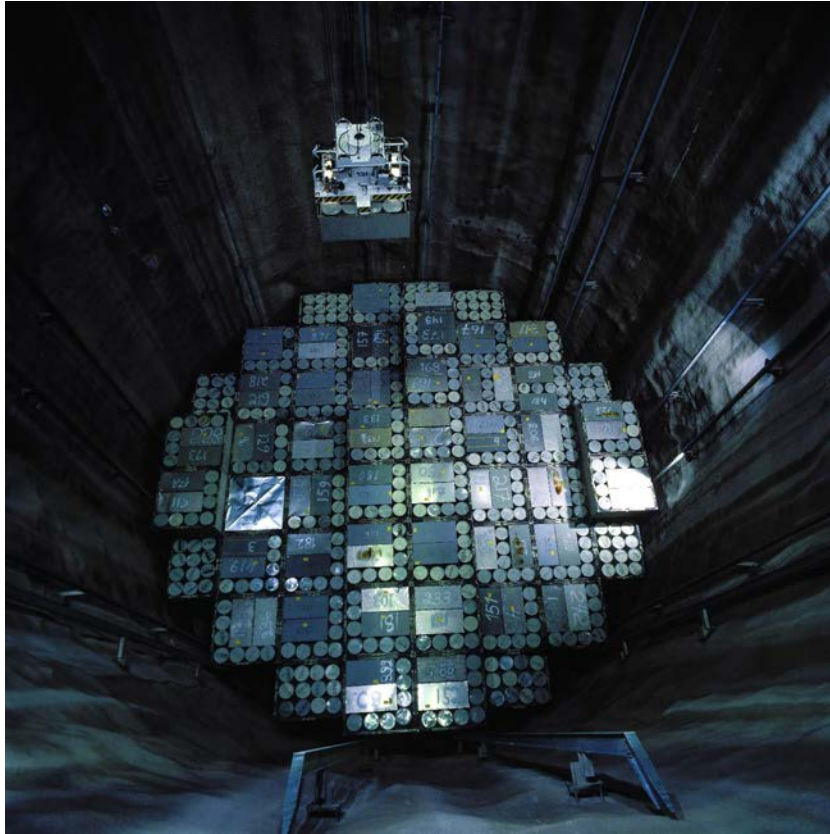
FIG. 13. Low level waste disposal facility in Olkiluoto, Finland (courtesy of TVO).
