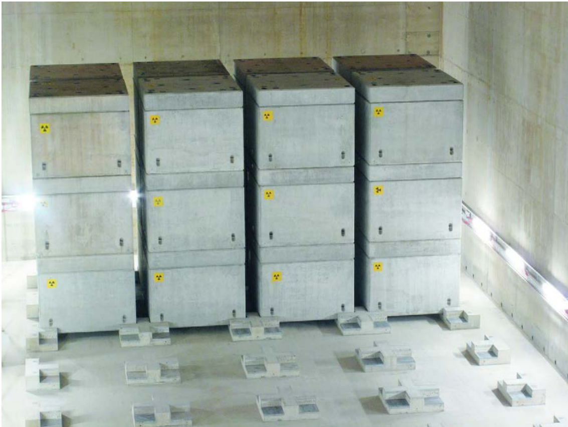
FIG. 16. Intermediate level waste storage at Trawsfynydd nuclear power plant, United Kingdom (courtesy of Nuclear Decommissioning Authority).
