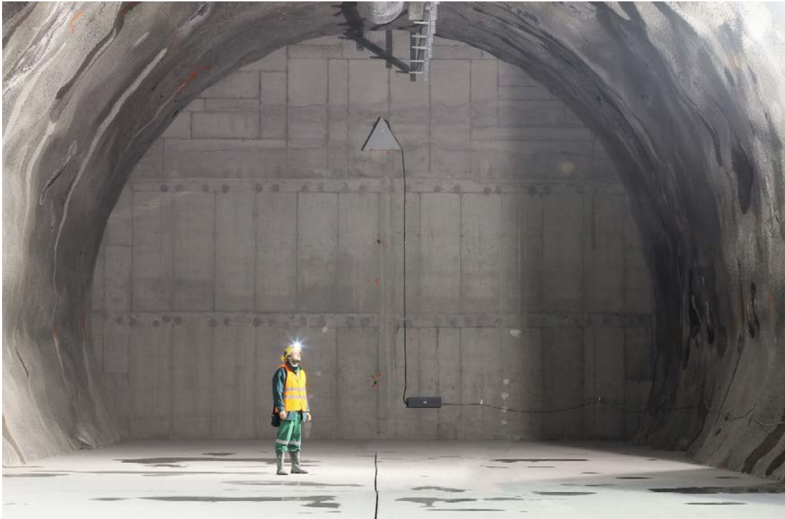
FIG. 15. Low and intermediate level radioactive waste disposal vault in Bataapati, Hungary (courtesy of PURAM).
