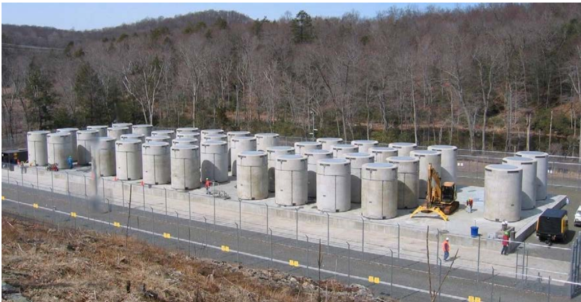
FIG. 8. Concrete casks storing spent fuel at the Connecticut Yankee nuclear power plant site (courtesy of NAC International).
