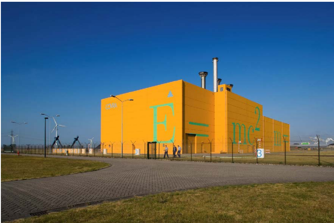
FIG. 12. Long term interim storage in the Netherlands (courtesy of COVRA).
