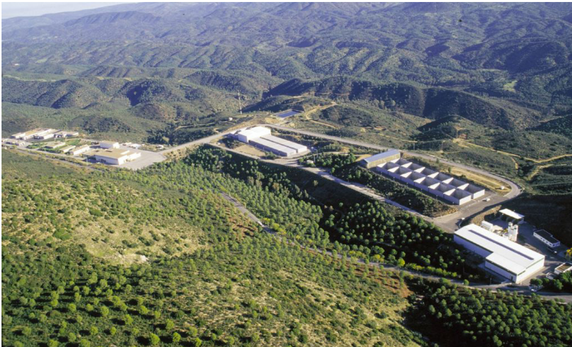
FIG. 14. Low level waste disposal facility in El Cbril, Spain (courtesy of Enresa).
