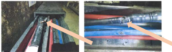
Point of interface power line (Normally 22.9kV line)
