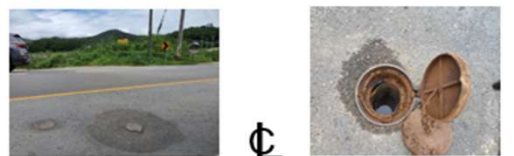
Manual water drain valve construction (past)
