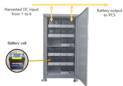
Battery and BMS Subsystem
