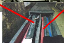
Point of interface power line (Normally 22.9kV line)
