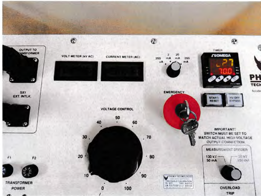
Test voltage – 15 kV
