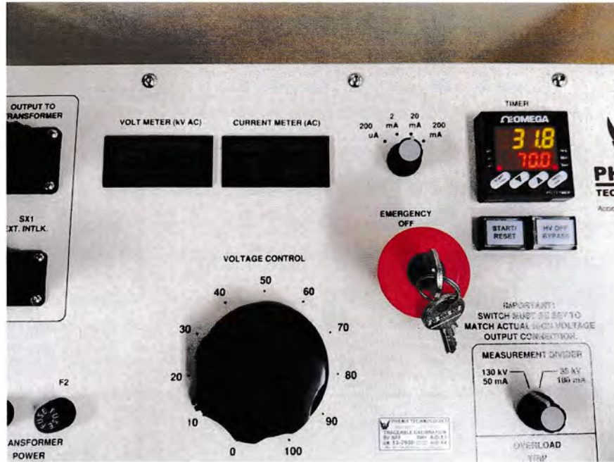
Test voltage – 20 kV
