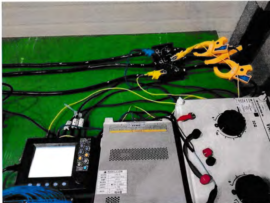
Track voltage/current measurement
