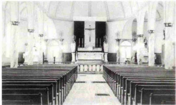
Interior of St. Agatha's First church Destroyed by fire August 13, 1940.
