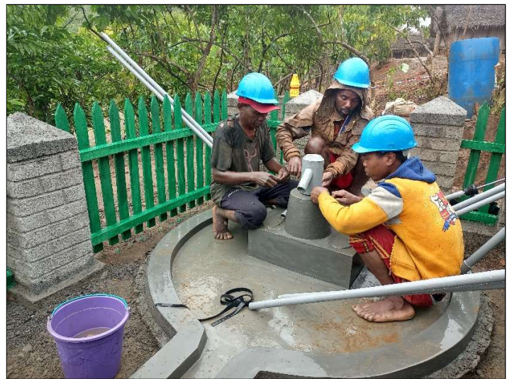
Practical training of local maintenance technicians on handling and assembly of the Canzee hand-pump.
