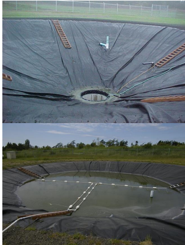
P-6.4: Anaerobic Pretreatment Cell
