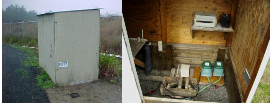
P-6.2: Influent Flow Meter and Building
