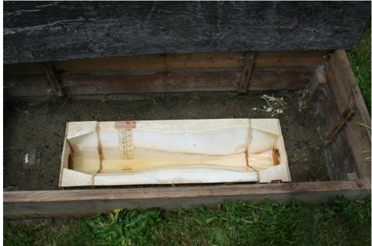
P-6.10: Plant Effluent Flume
