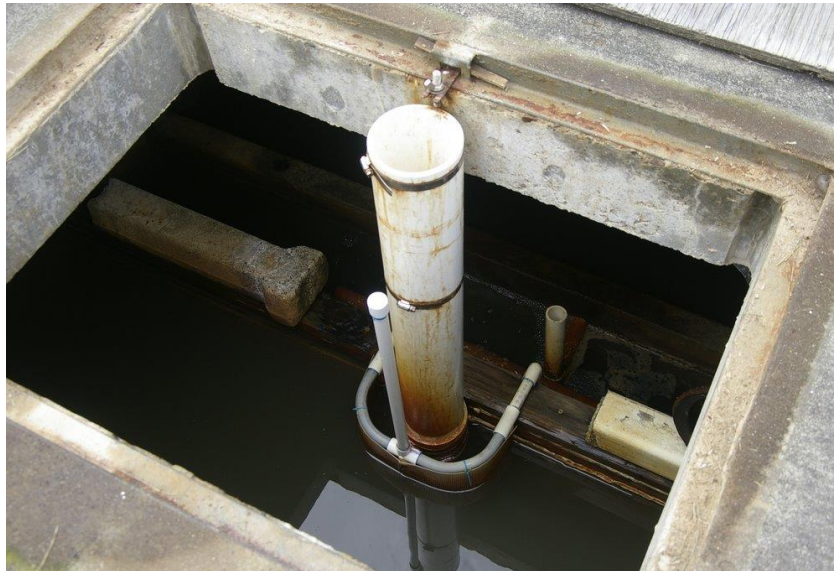
P-6.9: Chlorine Feed Device
