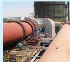
Sponge Iron Plant
