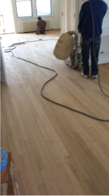
REPAIR AND REFINISH FLOORING
