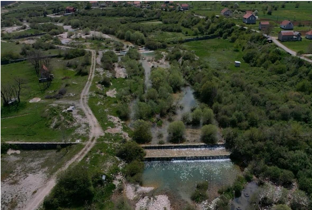
Identified barriers on Gračanica, upper Zeta basin
