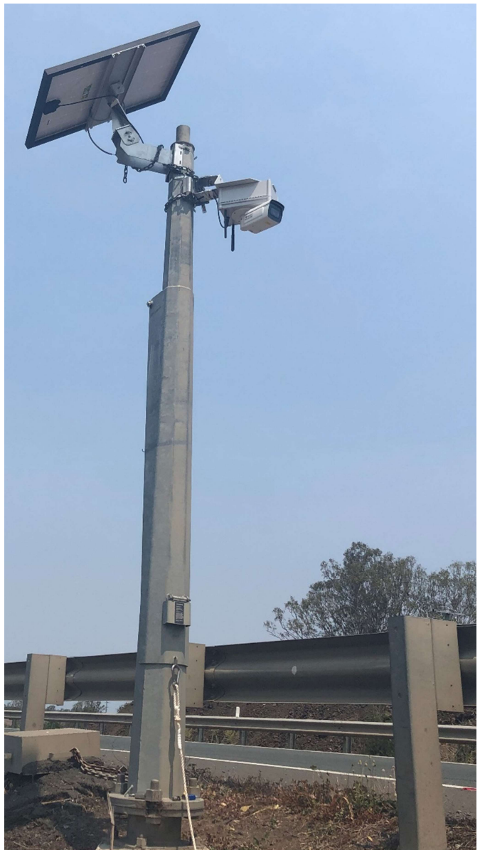
Temporary setup on existing TMR Pole for Trial
