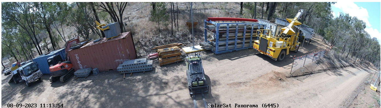
180° Plant & Equipment Monitoring - Day
