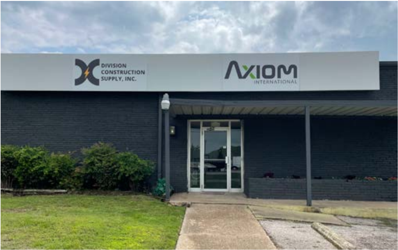
Headquarters Point, TX
