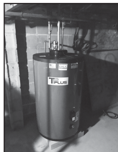
Hot Water Heater
