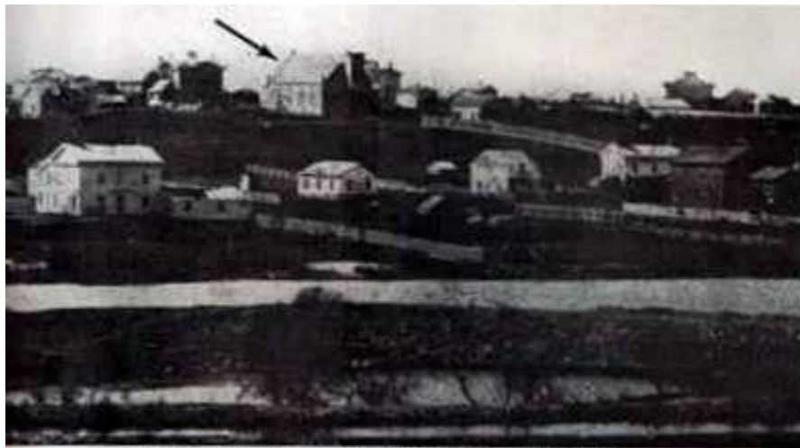
Original Trinity Episcopal Church, North Lake Street at Spruce Street, built 1884.
