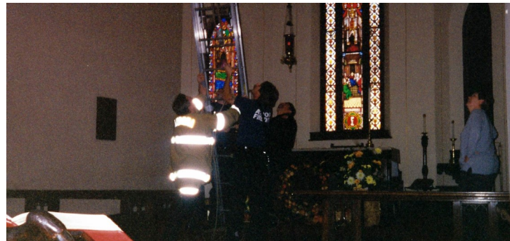
Firefighters replacing lights at the Altar
