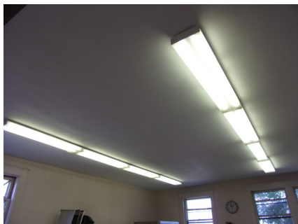
Kitchen Ceiling Painted
