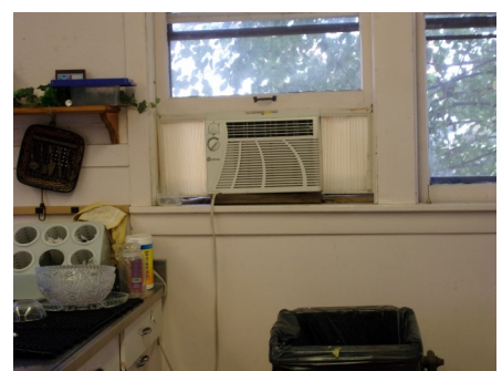
Cooling for the Kitchen
