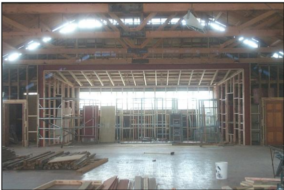
Steel posts and beams:... around the stage
