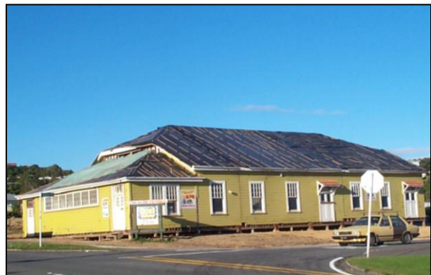
The three sections joined back together
