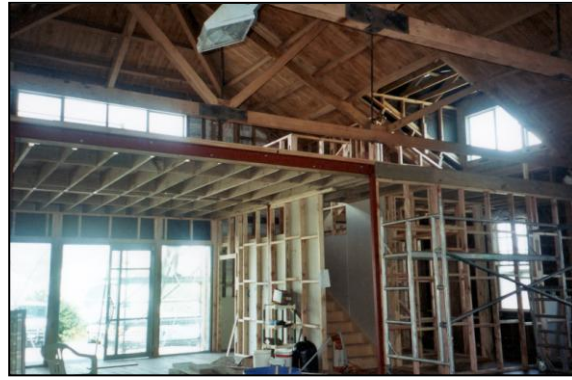
Steel posts and beams supporting upstairs
