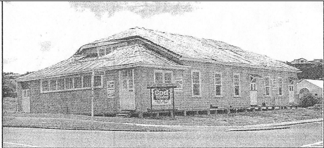
Maungaraki Baptist Church plans to upgrade this former dance hall.
