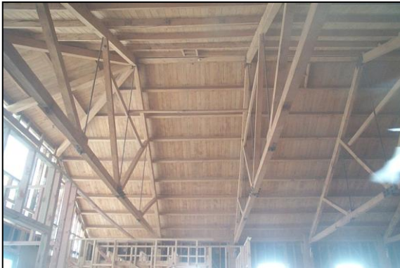
The Rimu ceiling after sand blasting
