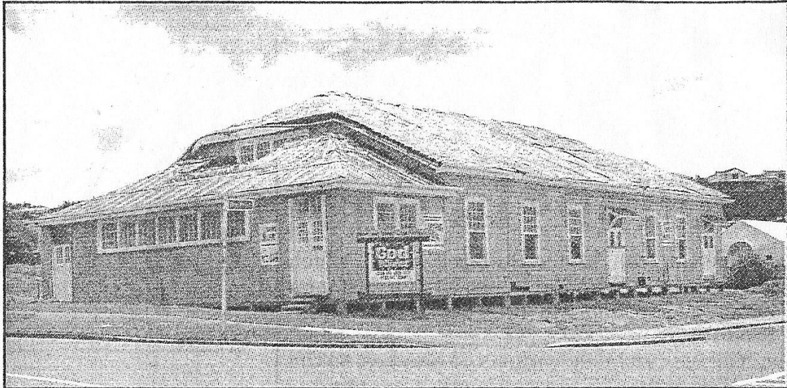
Maungaraki Baptist Church plans to upgrade this former dance hall.
