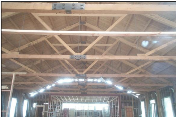
The sandblasted ceiling with up lighters on
