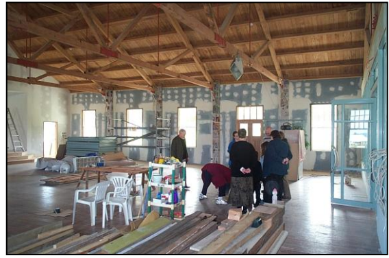
Walls GIB stopped and ready for painting
