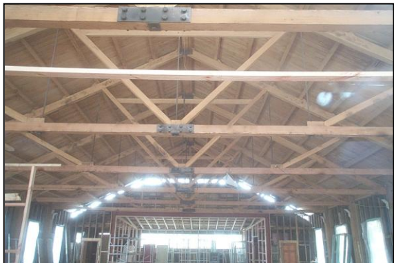
The Rimu ceiling and Oregon beams
