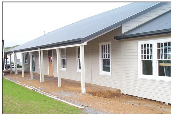
The verandah before the conservatory was constructed by MMM
