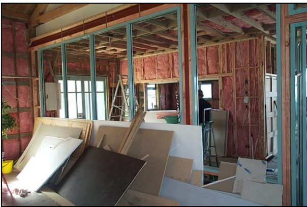
Starting to fix the GIB board
