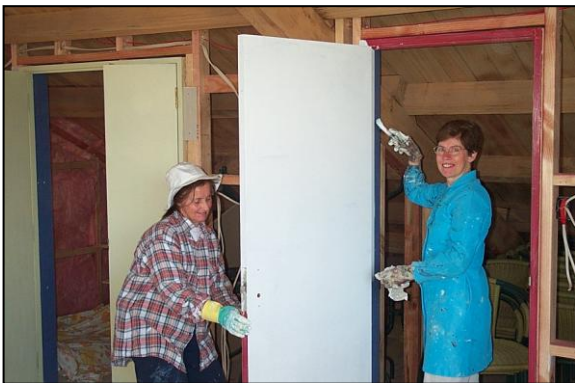
Fiona Coughlan and a volunteer from Hope Centre painting the doors upstairs. On the right, one of the original doors after being stripped and polyurethaned.
