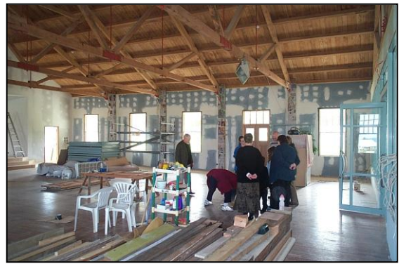
Walls GIB stopped and ready for painting
