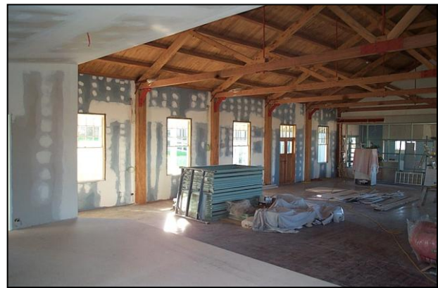
The GIB stopping completed, ready to paint
