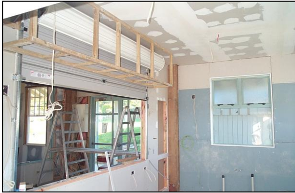
Kitchen in progress, roller door installed
