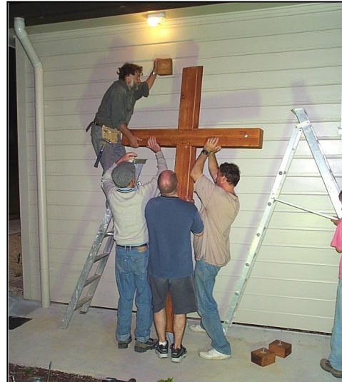
Fixing the cross to the building
