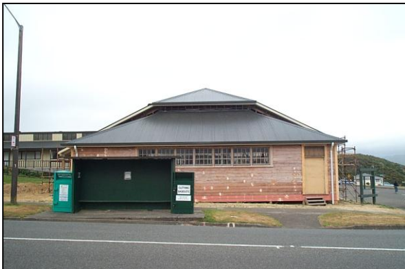
The bus shelter before it was moved ....
