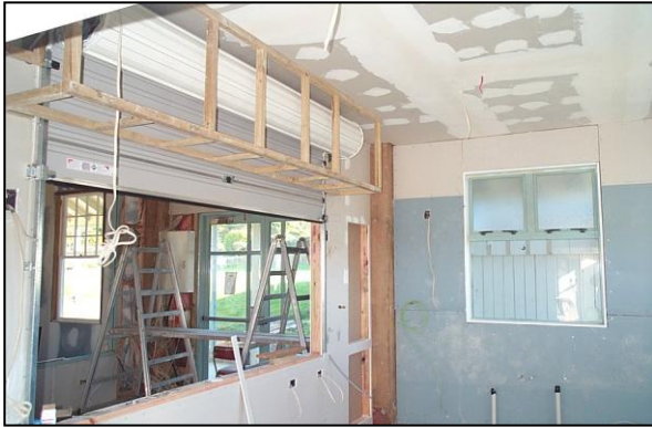
Kitchen in progress, roller door installed
