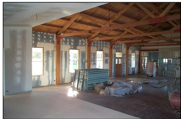
The GIB stopping completed, ready to paint
