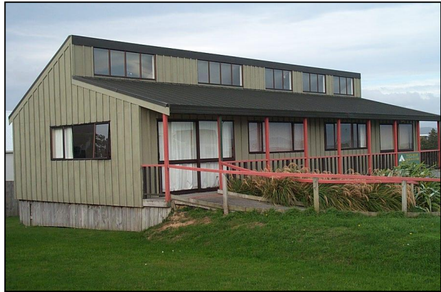
The Administration Building in 1995
