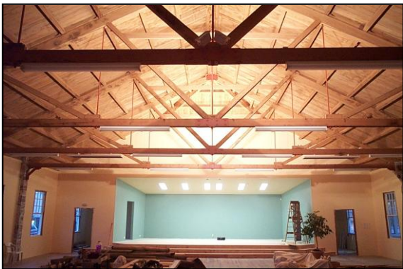
The sandblasted ceiling with up lighters
