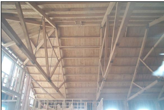
The Rimu ceiling after sand blasting
