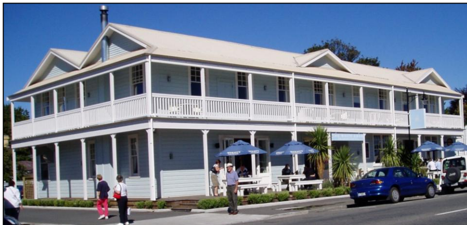
The Old Railway Administration Block is now the White Swan Hotel in Greytown
