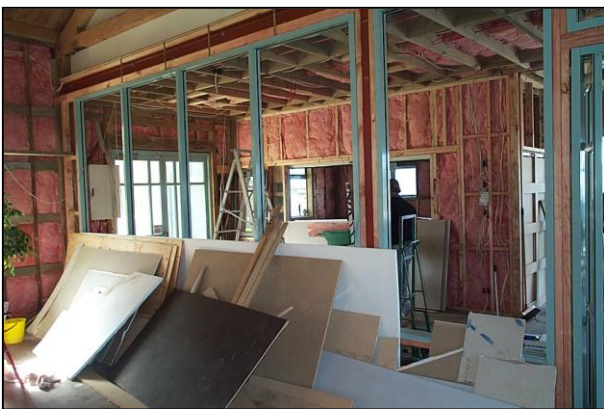
Starting to fix the GIB board
