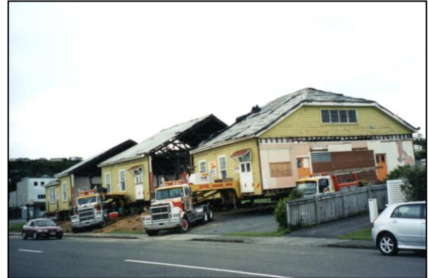
The three sections were in place on the Church land by 10.00 am 24 November 2002
