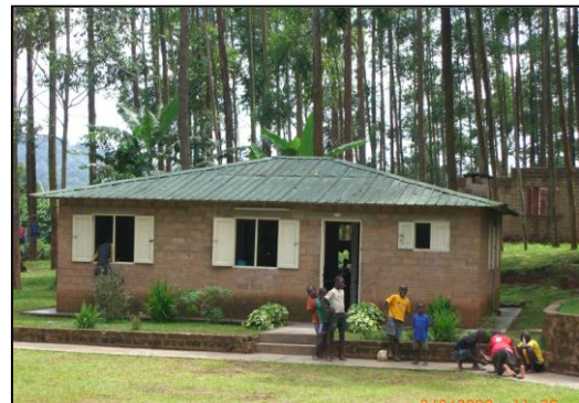
A finished home at Watoto village
