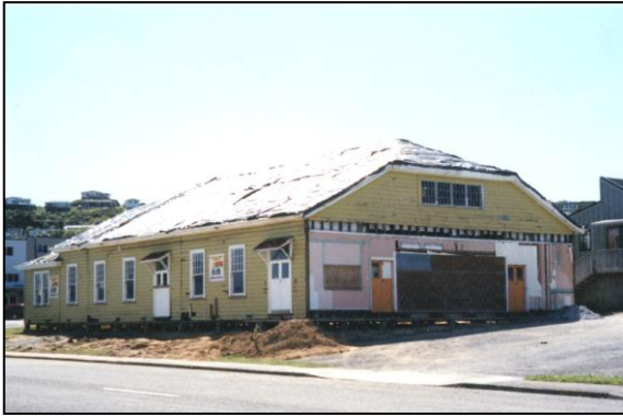
The wall that needed to be re-built
