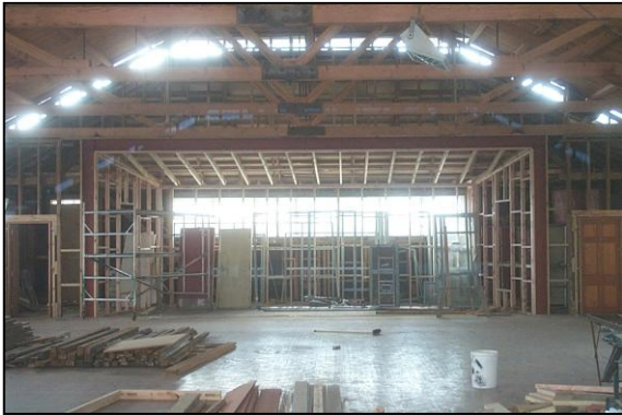
Steel posts and beams around the stage
