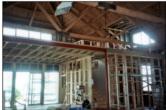
..... and supporting the upstairs
