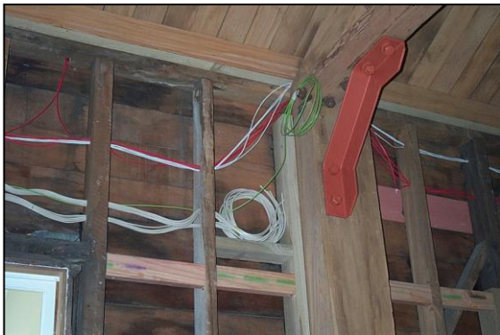
Cables pulled through the drilled holes
