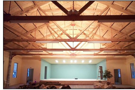
The Rimu ceiling and Oregon beams
