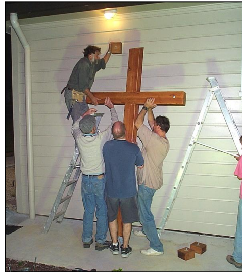
Fixing the cross to the building
