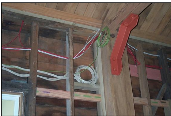
Cables pulled through the drilled holes
