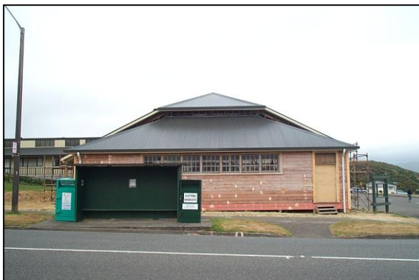
The Bus shelter before it was moved ....
