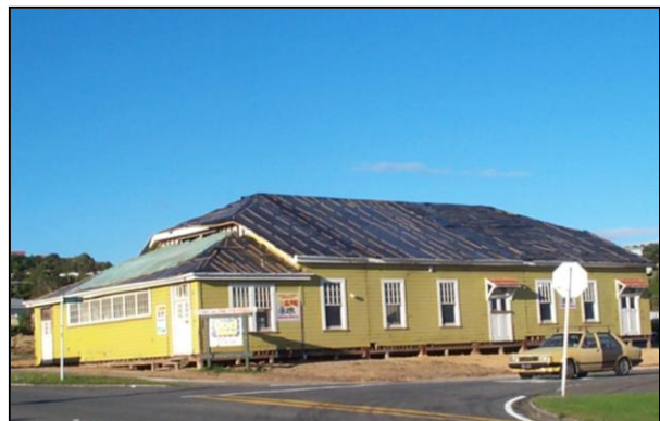
The three sections joined back together
