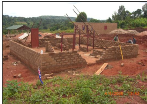
The Watoto home being built
