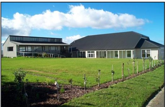
Both buildings are completed
