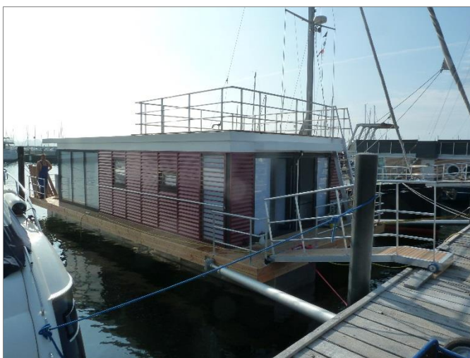
Floating home at the berth after commissioning of the BUSSE-MF
