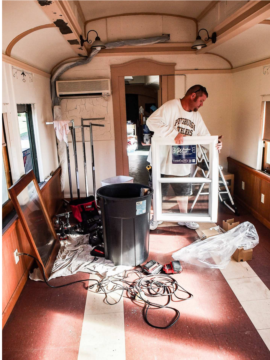
A worker for Window World of Pittsburgh installs a new window.
