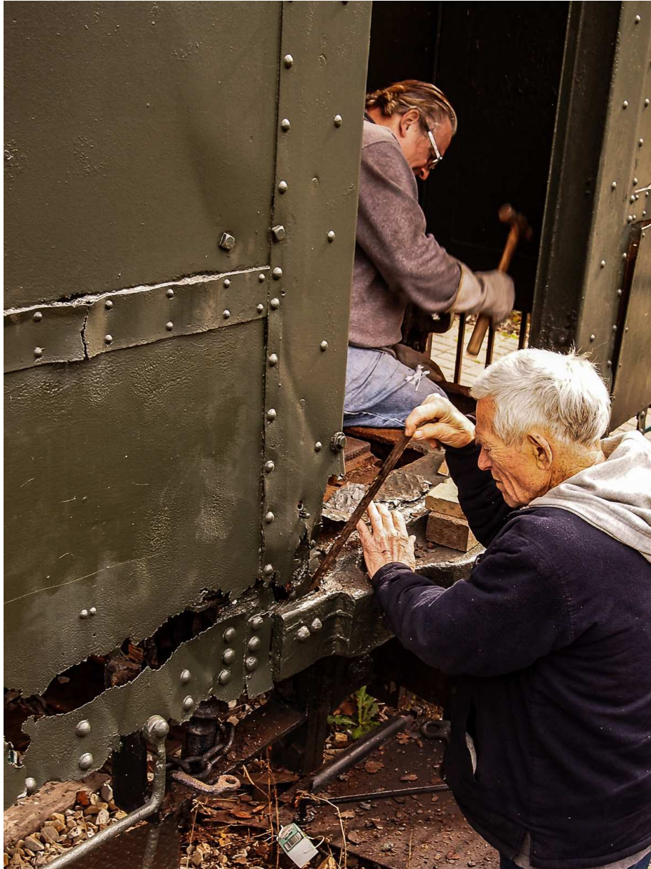
Chuck and Joe Wadsworth repair rust spots at the rear door.
