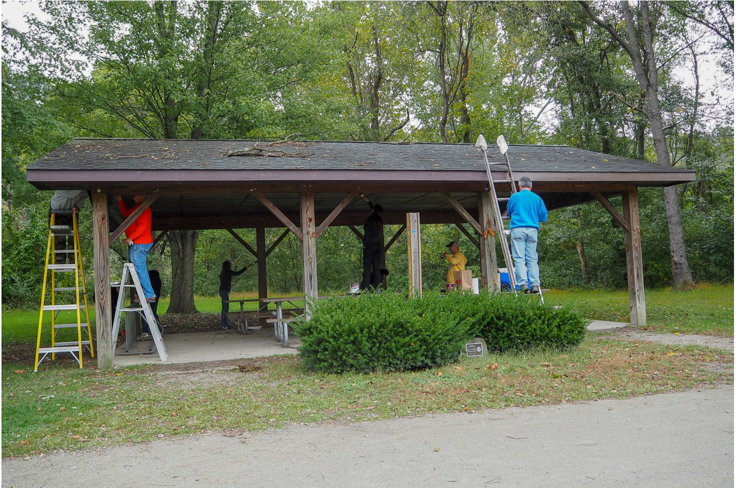
Club members each year perform maintenance on the pavilion.
