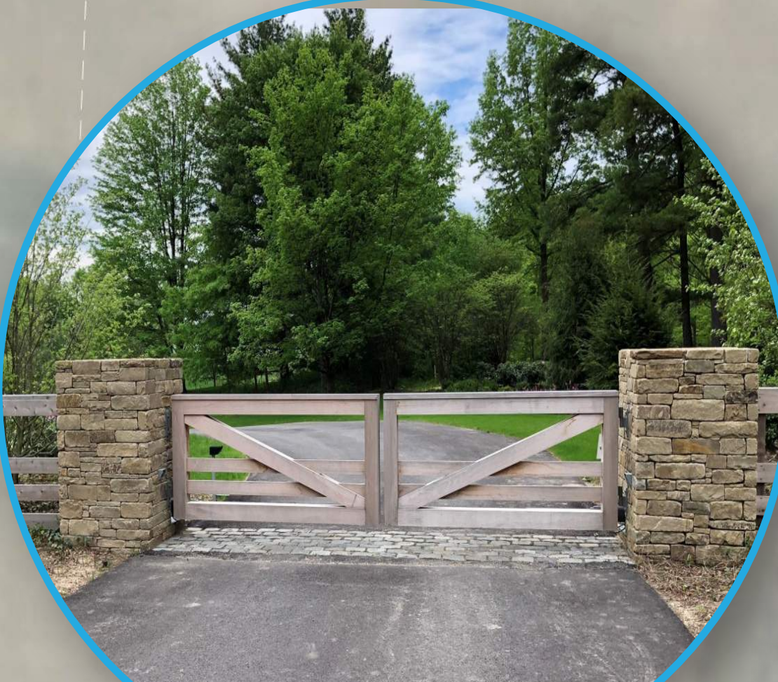
ENTRY PIER & GATES
