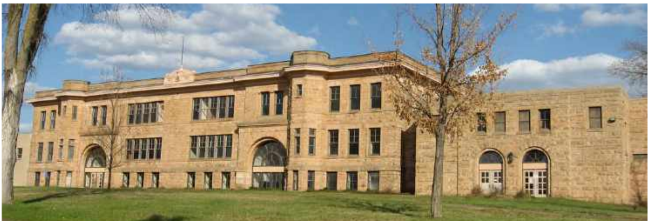
Figure 2: School building in Sandstone, Minnesota [Photograph]. Kathy George, 2018.
