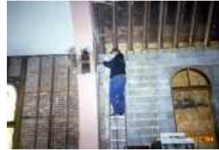
Figure 24: Volunteers working on the Red Rock center restoration [Photograph] Red Rock Center, 2018.
