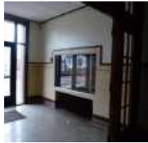
Figure 45 : Emerson School Entrance [Photo]. Community Housing Development Corporation, 2018.
