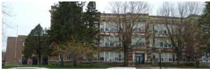
Figure 43 : Emerson School Entrance [Photo]. Community Housing Development Corporation, 2018.
