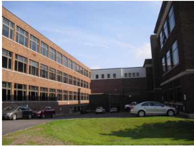
Figure 9: Cloquet Middle School building. [Photograph]. Holly Hansen, 2018d.
