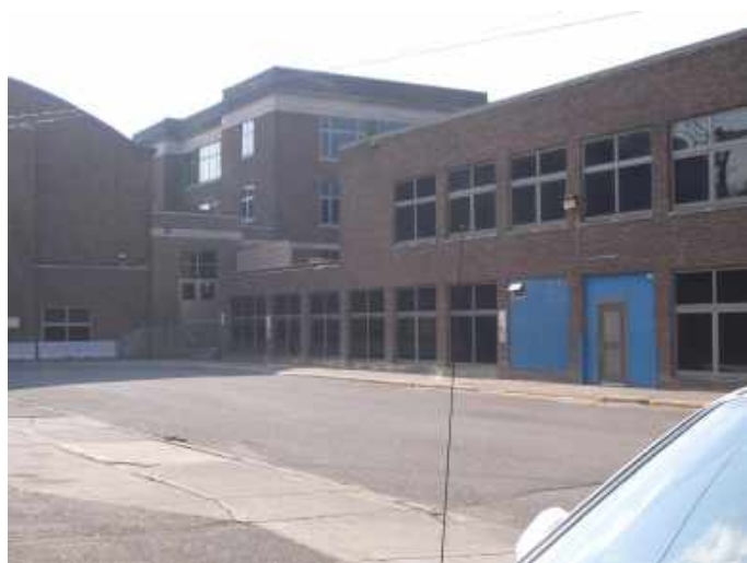
Figure 7: Cloquet Middle School building. [Photograph]. Holly Hansen, 2018b.
