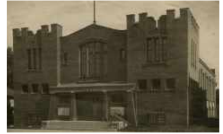
Figure 56 : St. Peter Armory [Photo]. Nicollet Co. Historical Society, 1918.
