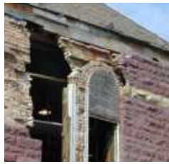
Figure 22: Red Rock Center exterior damage [Photograph]. 2018.
