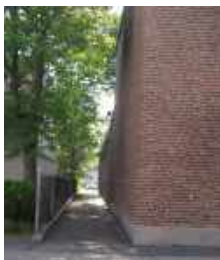
Figure 8: Cloquet Middle School building. [Photograph]. Holly Hansen, 2018c.
