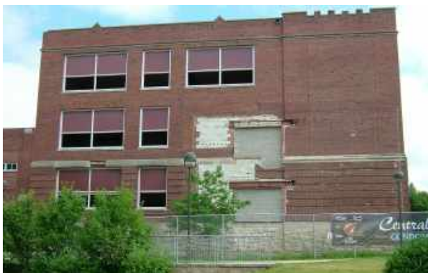
Figure 53 : Central High School exterior damage [Photo]. City of Red Wing, 2003.
