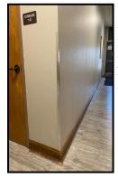
Aluminum corner moldings were installed to protect corners in the hall-ways from bumps and bruises.
