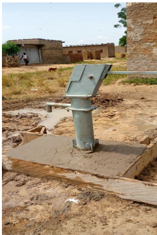
Cemented base borehole
