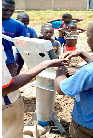
Pump Head Installation
