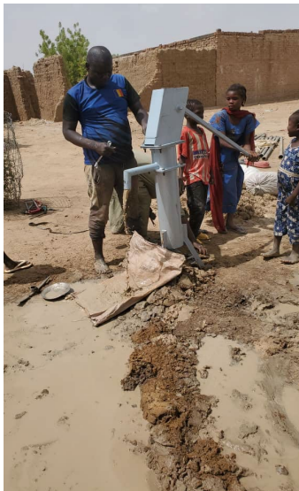
Installation of the pump head
