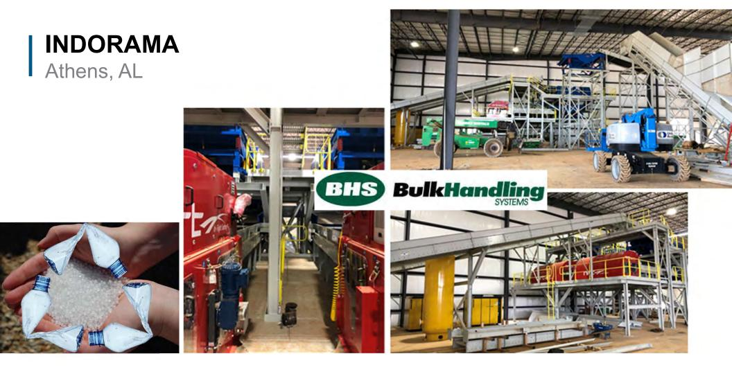
Project: Plastics recycling process line plant expansion Description: Installation of cleaning, sorting, and sizing equipment Contract: Lump Sum
