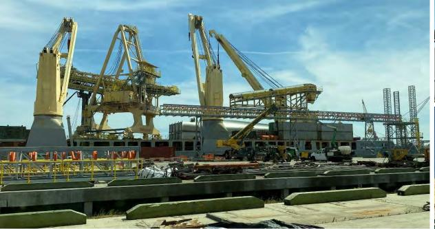
Project: Wood pellet export facility Description: Installation of a Ship Loader and Conveyors
