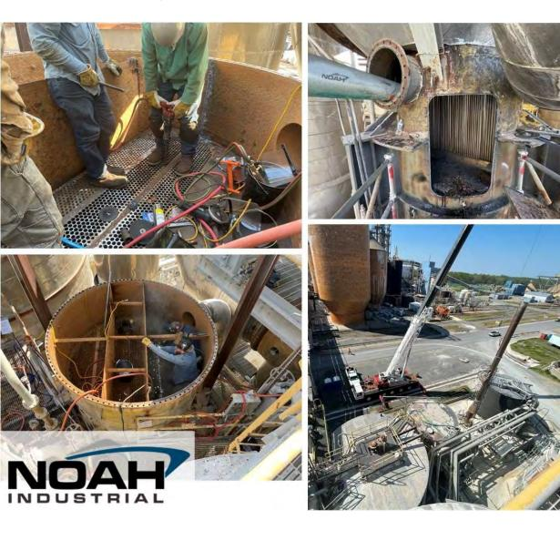
Project: Surface Condenser Retube Description: Installation of 2,500 new stainless tubes Contract: Lump Sum Completion: April 2021
