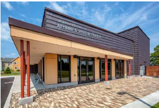
Back Entrance into the Multi-Purpose Room
