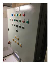
A customer had a problem wherby their PLC in their steering control system had a number of issues. The system consisted of a main control panel, bridge controls and wing controls located on the port and starboard wings respectively. A number of inputs had failed and the PLC was obsolete. Due to the condition of the aforementioned PLC and the run-down nature of the main panel, it was agreed that the panel should be replaced in its entirity.
