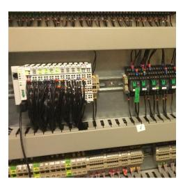
A customer had a problem wherby their PLC in their aft hydraulic control system had a number of issues. The panel controls the passarelle, stern door and lazarette crane. A number of inputs had failed and there were intermittent problems causing the crew to have to manually operate the hydraulics. Due to the condition of the aforementioned PLC and the run-down nature of the main panel, it was agreed that the panel should be replaced in its entirity.
